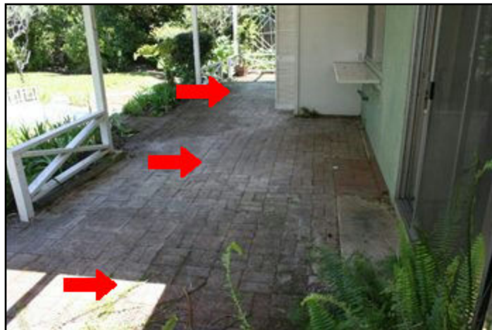
24. Slope toward house
