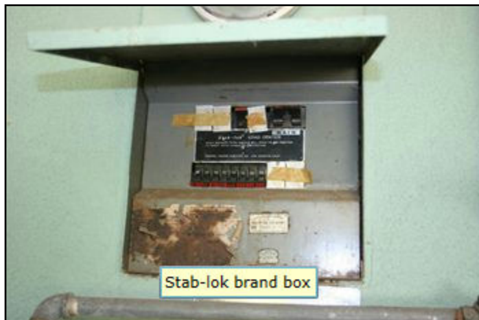
33. Obsolete service box
