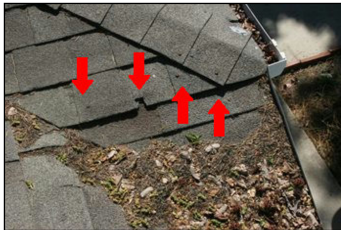
4. Exposed fasteners
