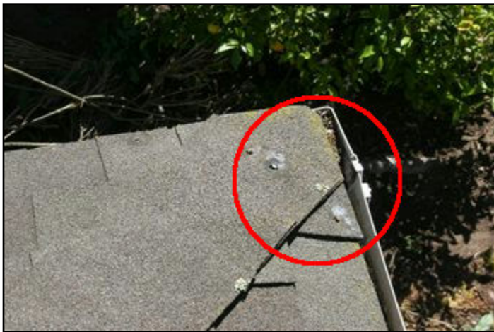
2. Exposed fasteners
