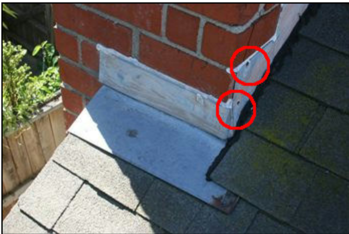
5. Damage, loose, open seams, patched
