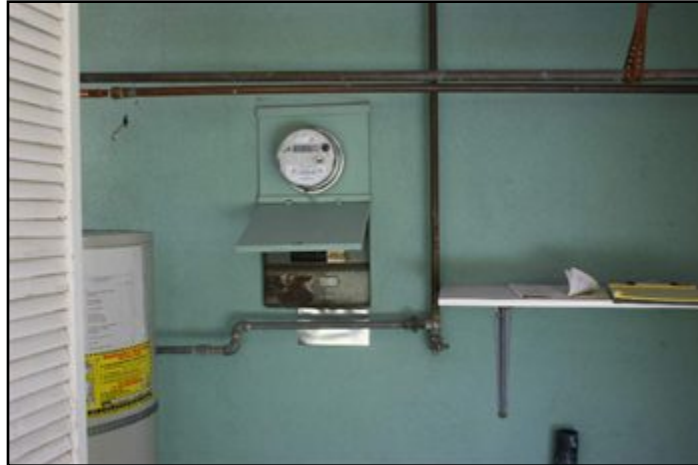
32. Breakers -exterior wall
