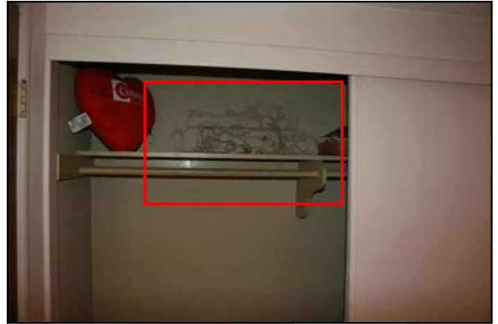
62. Evidence of termites
