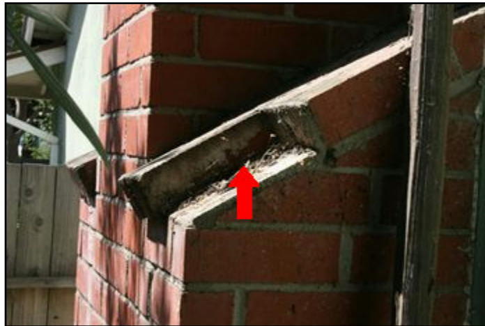
47. Loose, missing or deteriorated masonry
