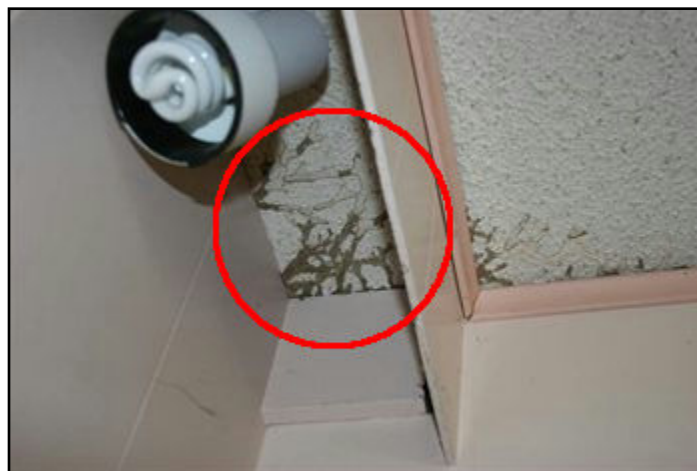
63. Evidence of termites
