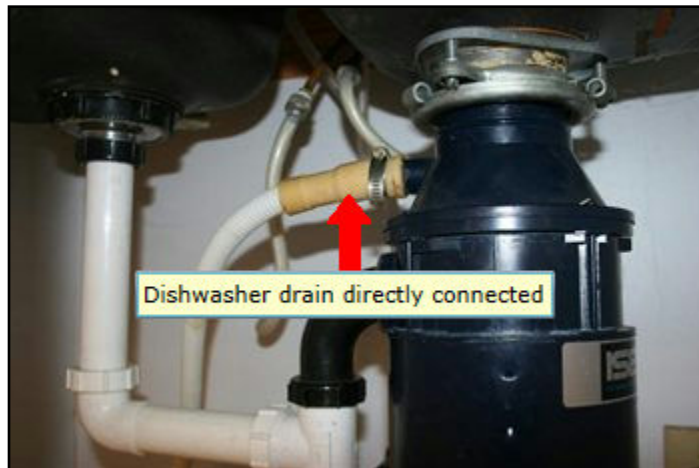
77. Backflow prevention missing
