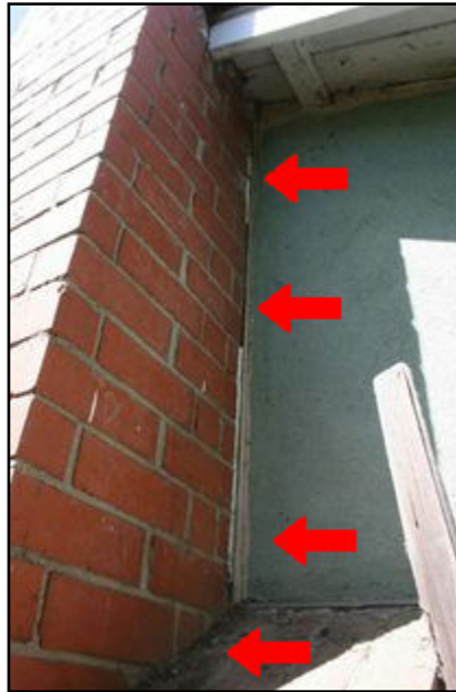
9. Damage, loose, open seams, patched
