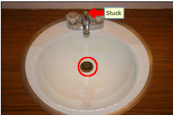
58. Drain stop ineffective
