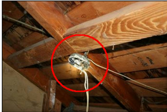
41. Cover loose or missing
