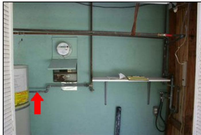
55. Inadequate support
