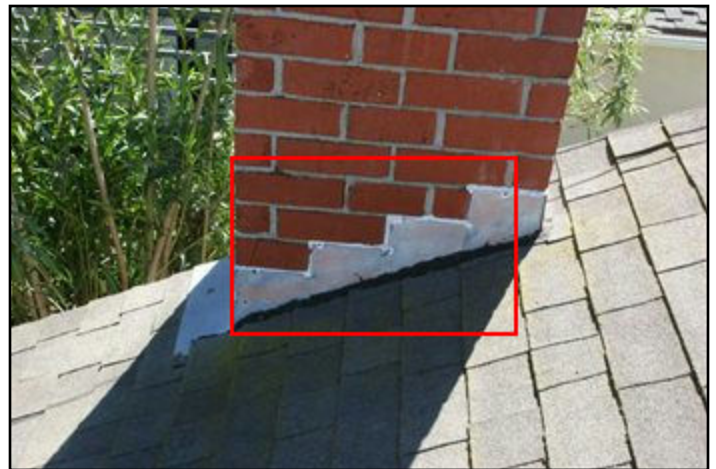
6. Damage, loose, open seams, patched
