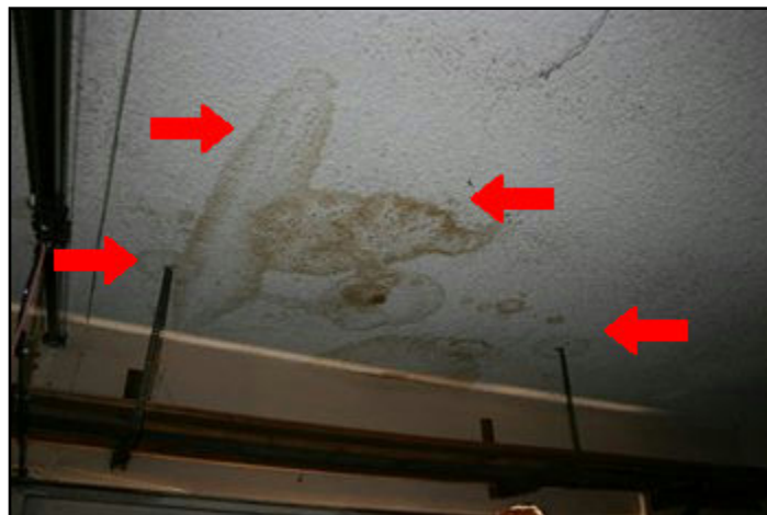
72. Evidence of moisture
