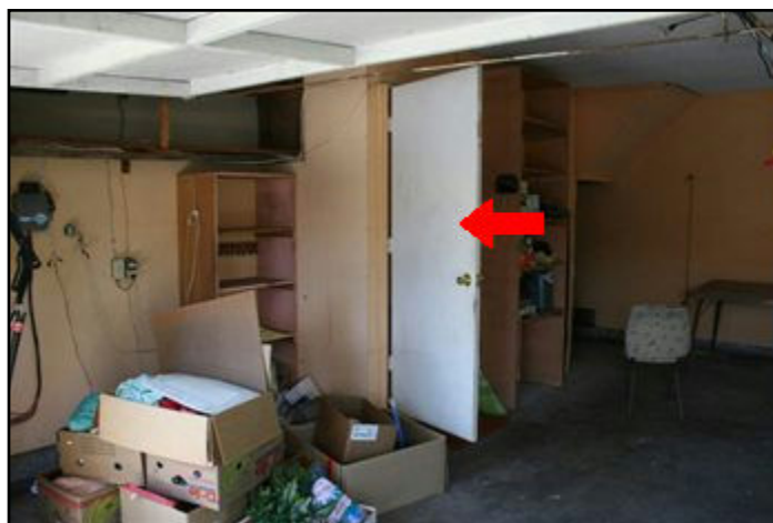
73. Door not fire rated or exterior type
