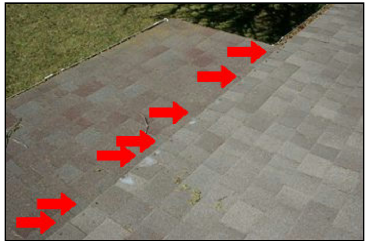
3. Exposed fasteners
