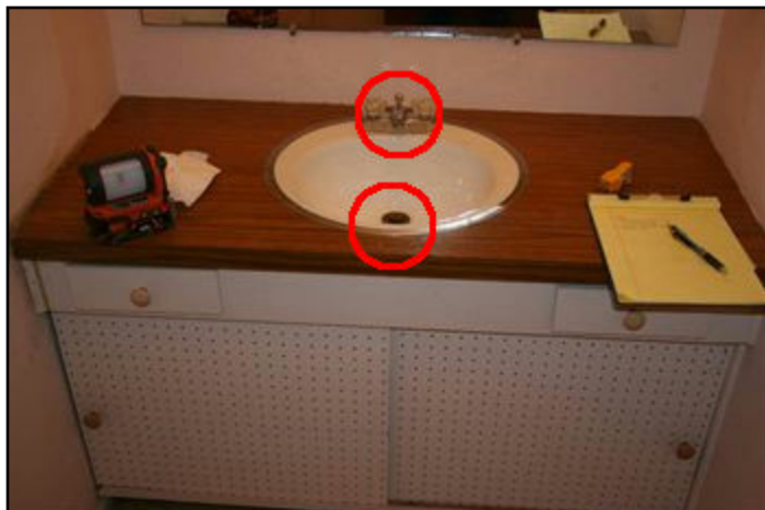
59. Drain stop ineffective
