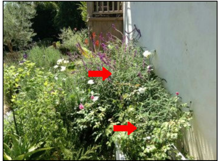
39. Trees or shrubs too close to house
