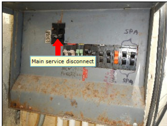
62. Breakers -exterior wall
