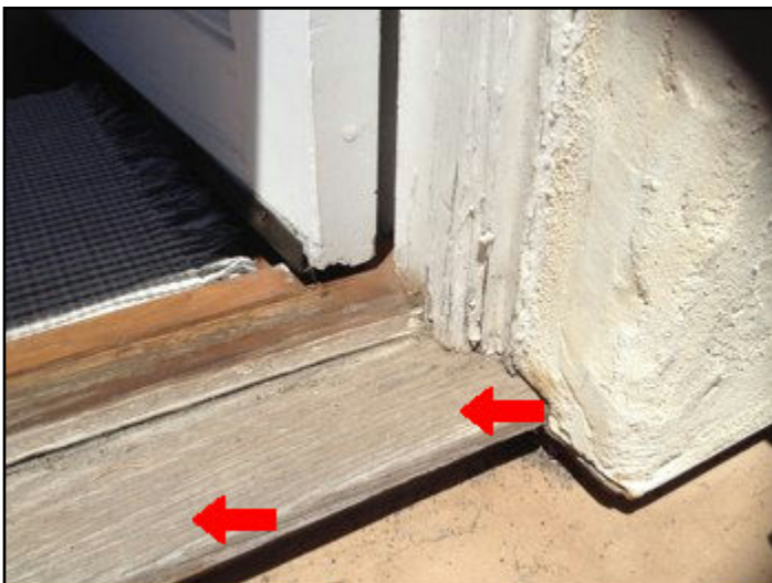
22. Paint or stain needed
