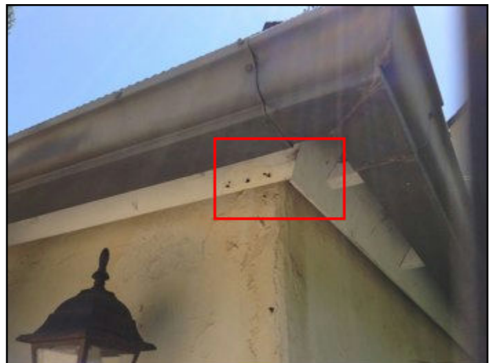
14. Rot or insect damage
