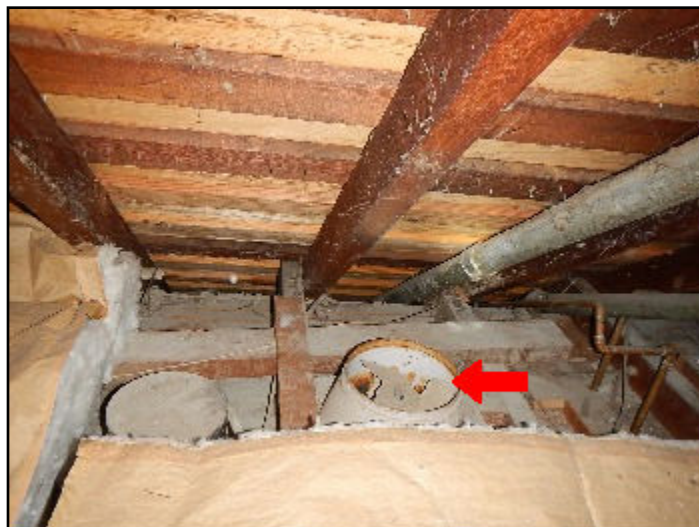
108. Not vented to exterior
