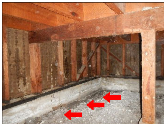
106. Dampness on floor or walls
