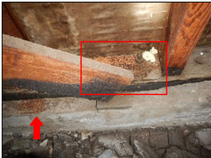
54. Rot or insect damage
