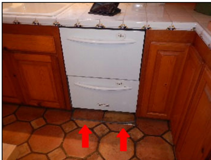
97. Grout missing
