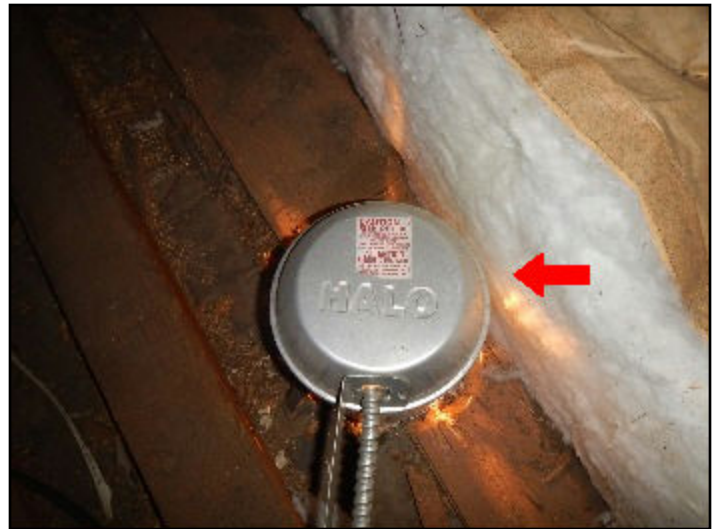
83. Covering can lights
