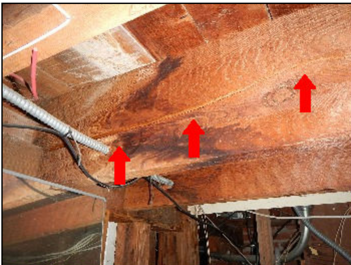
55. Split or damaged
