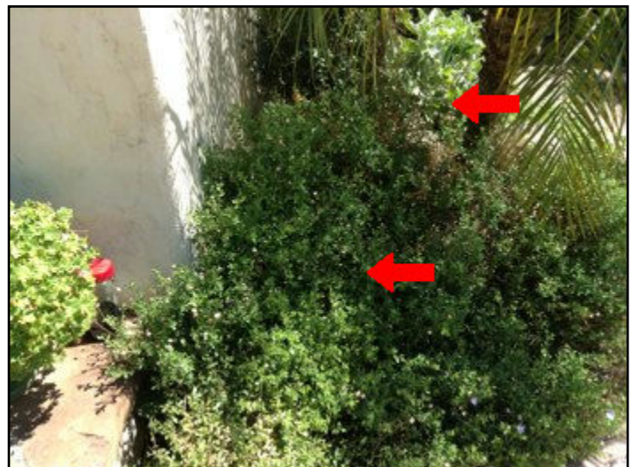
37. Trees or shrubs too close to house
