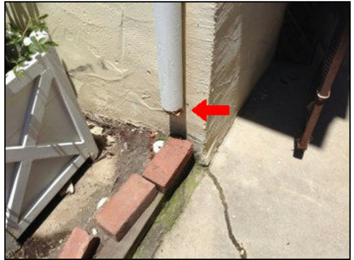
12. Downspouts end too close to building
