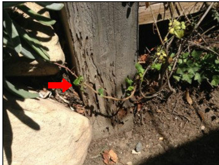
40. Rot or insect damage
