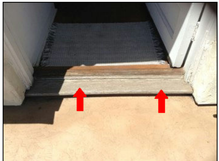
23. Paint or stain needed
