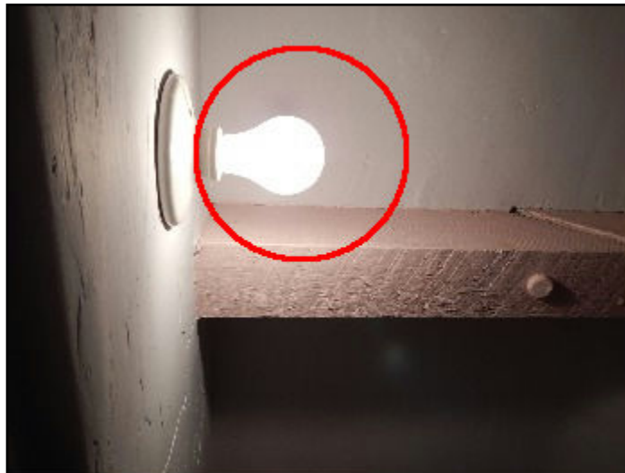
67. Improper closet lighting
