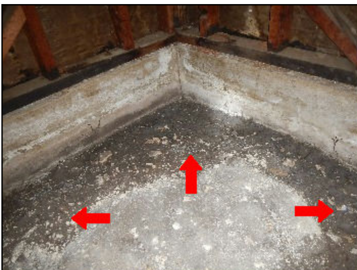
105. Dampness on floor or walls
