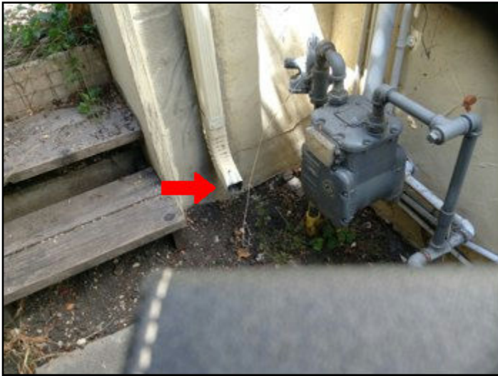
11. Downspouts end too close to building
