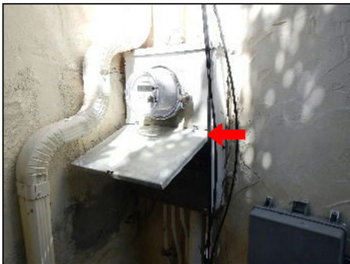
61. Breakers -exterior wall
