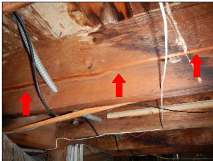
56. Split or damaged
