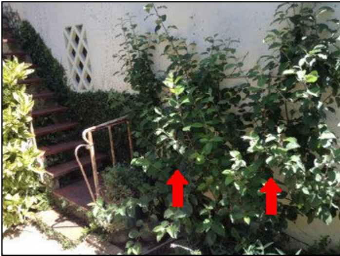
38. Trees or shrubs too close to house
