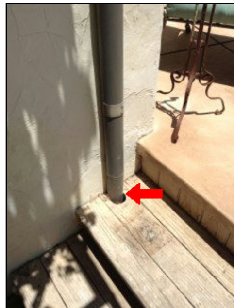
10. Downspouts end too close to building
