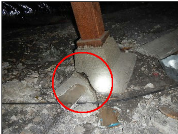
53. Mechanical damage
