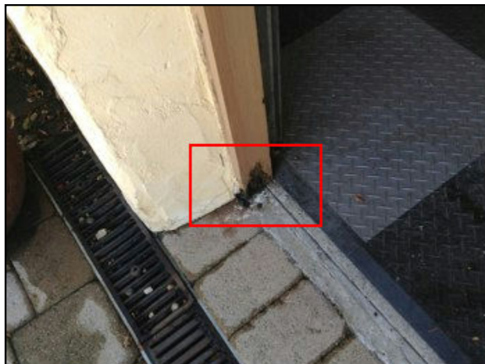
16. Rot or insect damage
