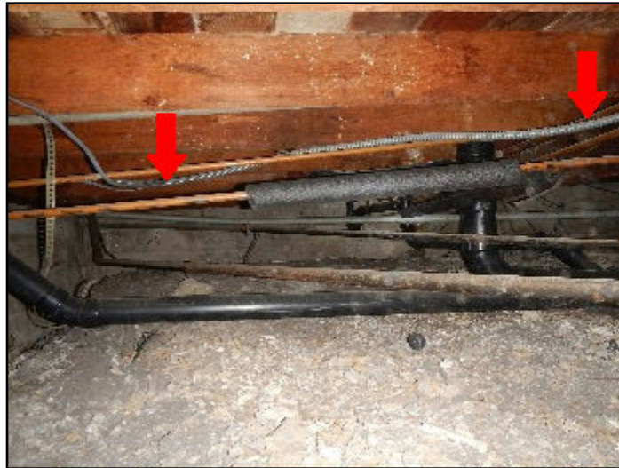
66. Not well secured
