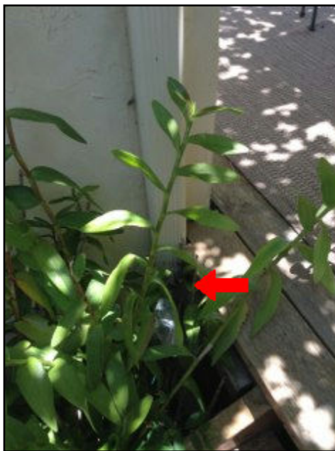
9. Downspouts end too close to building
