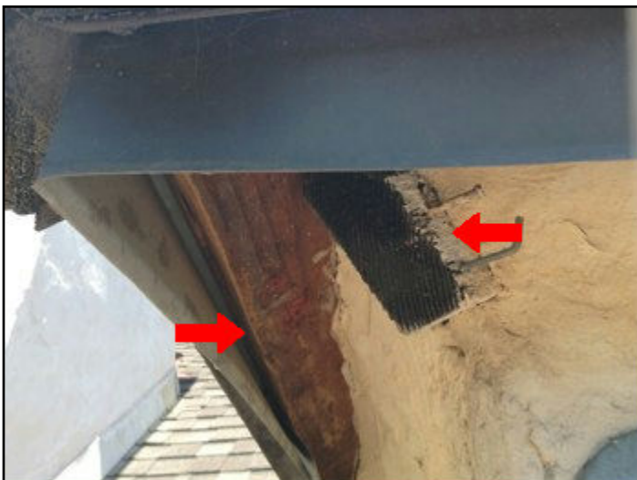
13. Rot or insect damage
