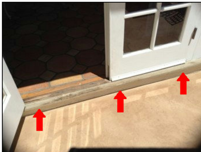
24. Paint or stain needed
