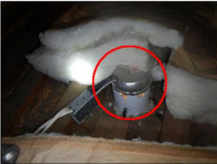
82. Covering can lights
