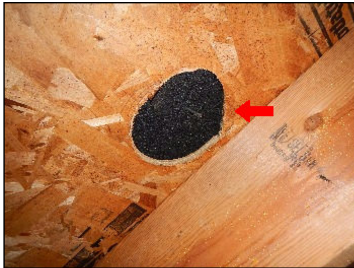
37. Hole in sheathing
