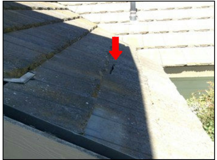
7. Missing, loose or broken pieces
