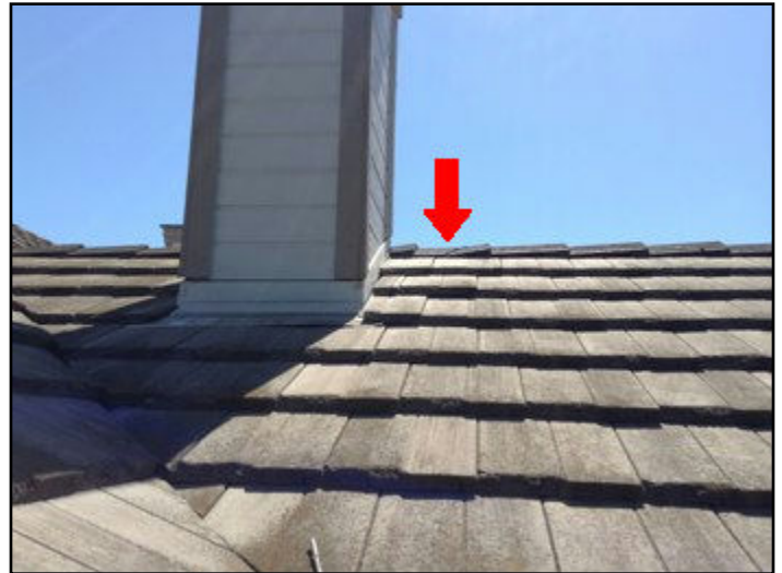
5. Missing, loose or broken pieces
