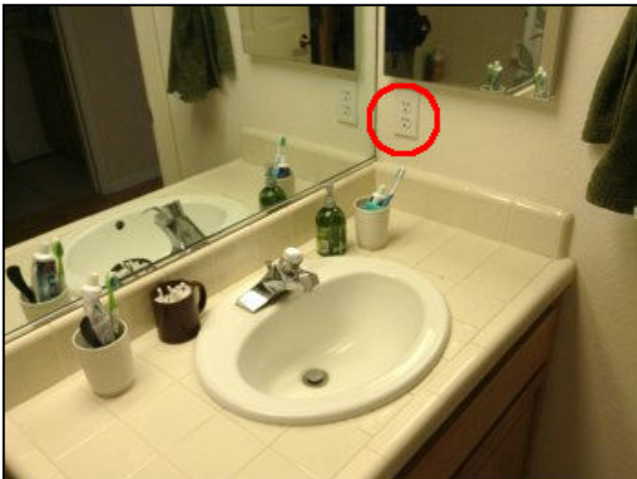
43. Ground Fault Interrupter (GFI) needed
