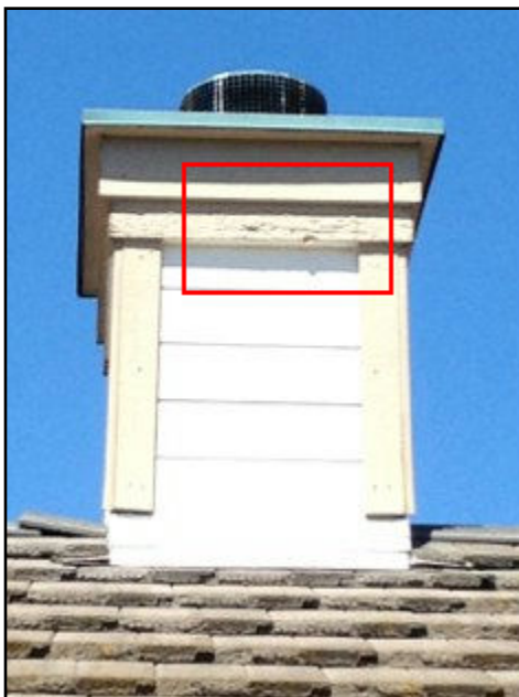
27. Rot or insect damage
