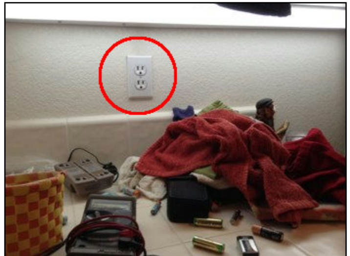
44. Ground Fault Interrupter (GFI) needed
