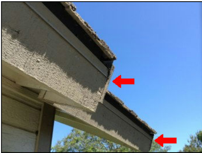
20. Rot or insect damage
