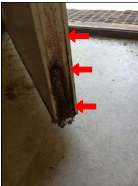
31. Rot or insect damage
