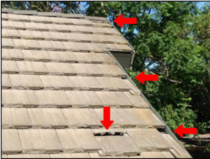
2. Missing, loose or broken pieces
