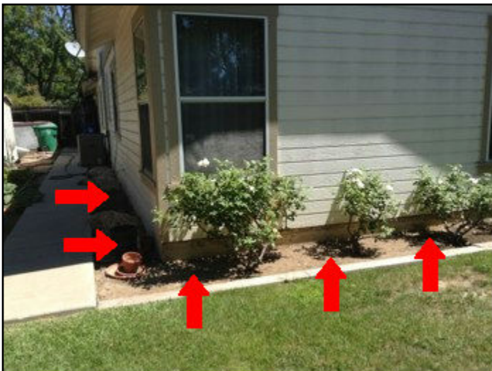
33. Improper slope
