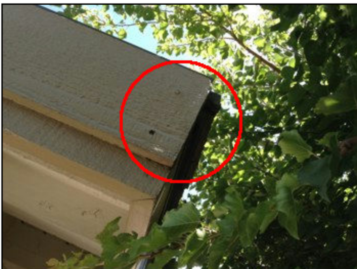
18. Rot or insect damage
