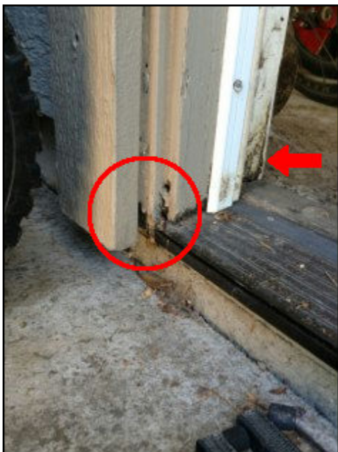
29. Rot or insect damage
