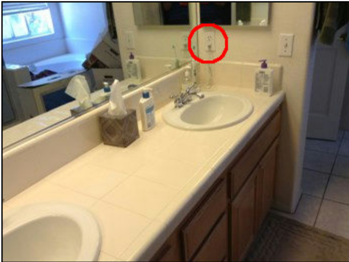
41. Ground Fault Interrupter (GFI) needed
