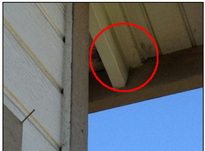
19. Rot or insect damage
