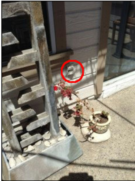
47. Ground Fault Interrupter (GFI) needed
