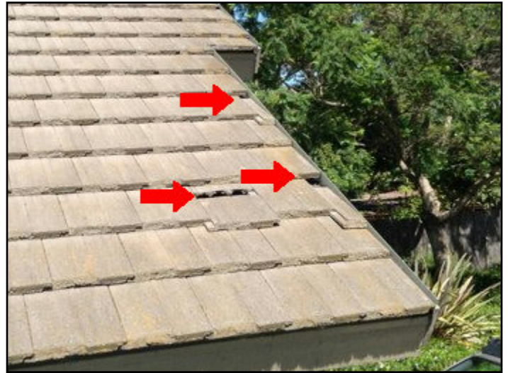
11. Missing, loose or broken pieces
