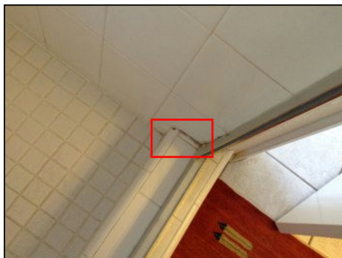
64. Caulking loose, missing or deteriorated
