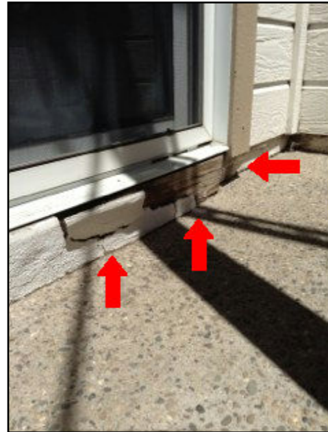
26. Rot or insect damage
