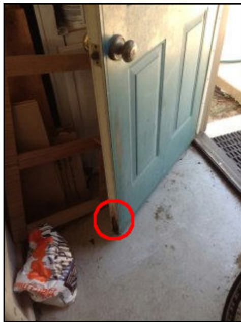
32. Rot or insect damage
