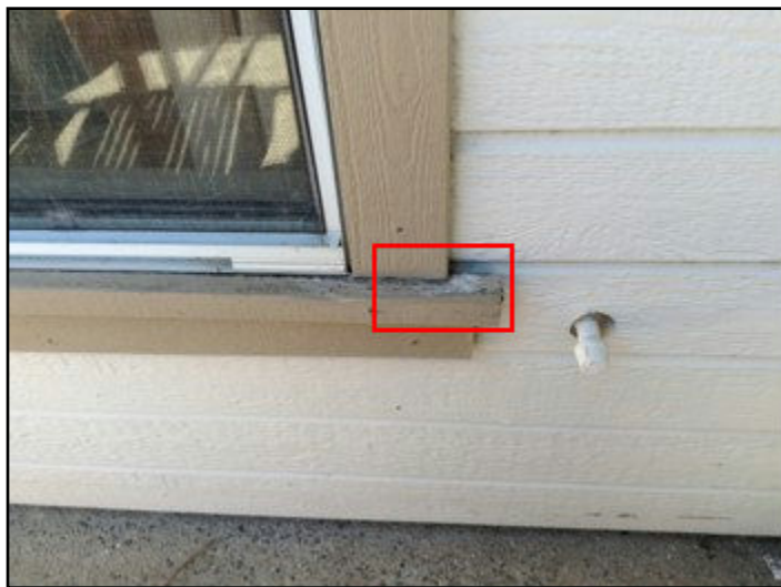
30. Rot or insect damage
