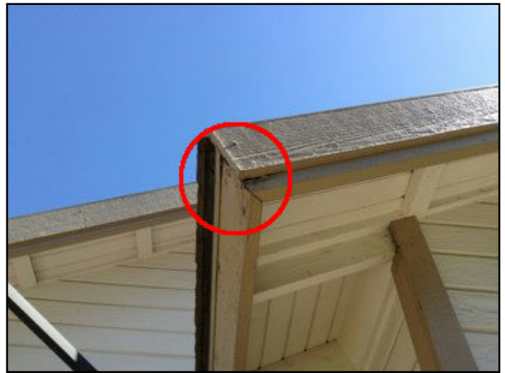
21. Rot or insect damage
