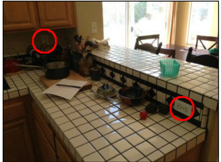
42. Ground Fault Interrupter (GFI) needed
