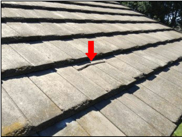
6. Missing, loose or broken pieces
