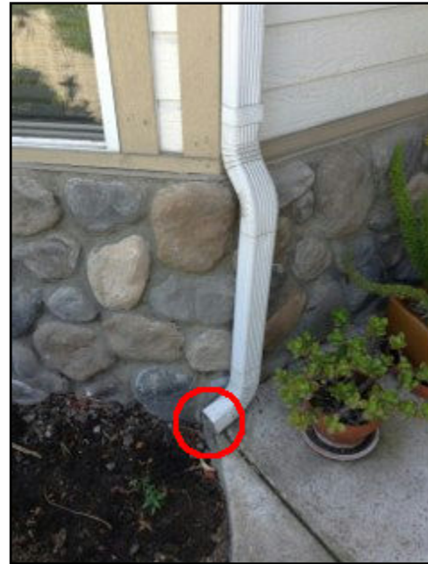
17. Downspouts end too close to building
