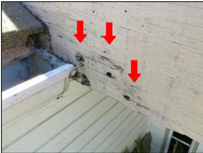
22. Rot or insect damage
