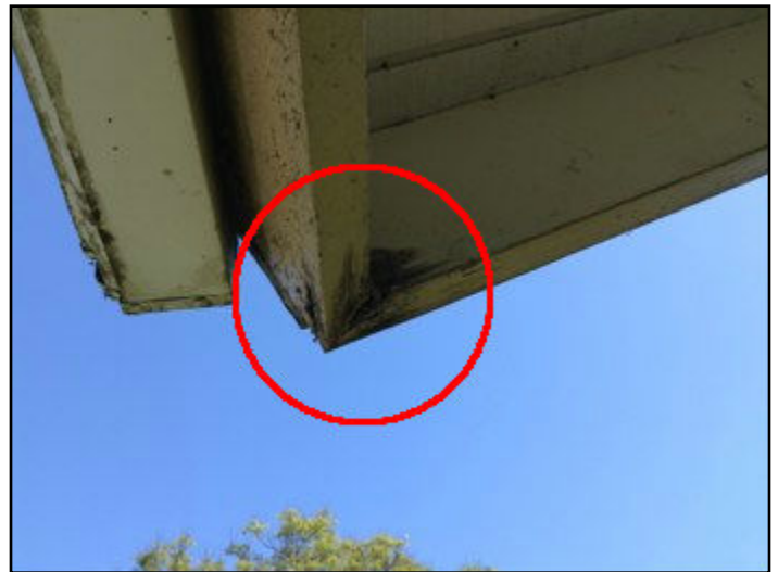
23. Rot or insect damage
