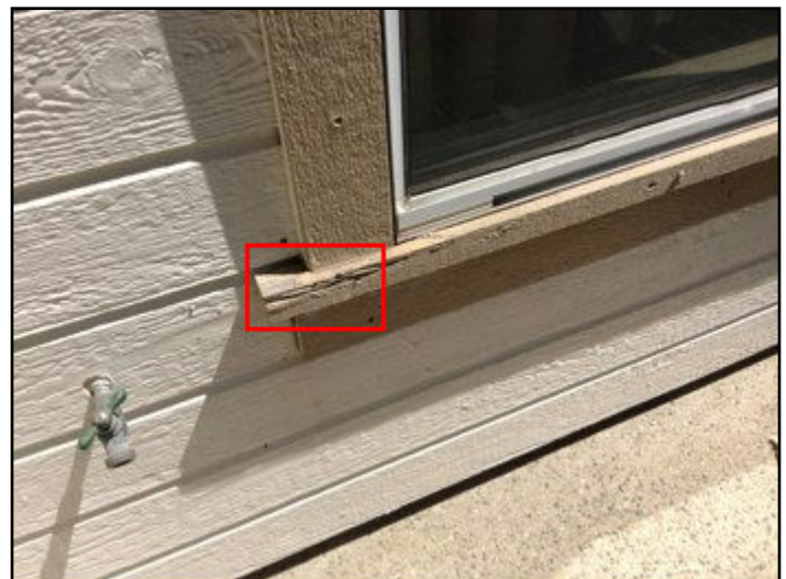
28. Rot or insect damage
