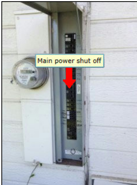
39. Breakers -exterior wall
