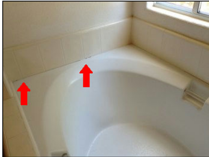
63. Grout loose, missing or deteriorated
