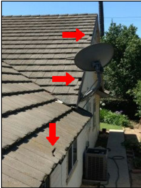
10. Missing, loose or broken pieces
