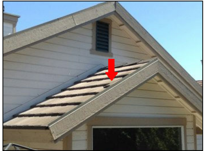
3. Missing, loose or broken pieces
