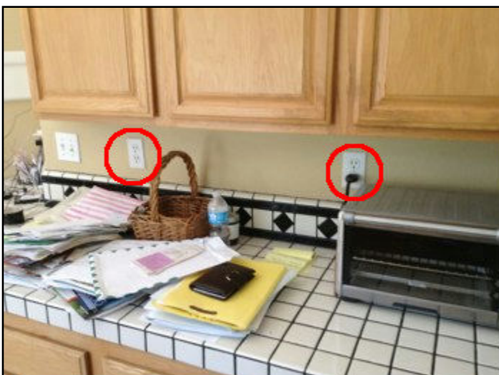
45. Ground Fault Interrupter (GFI) needed
