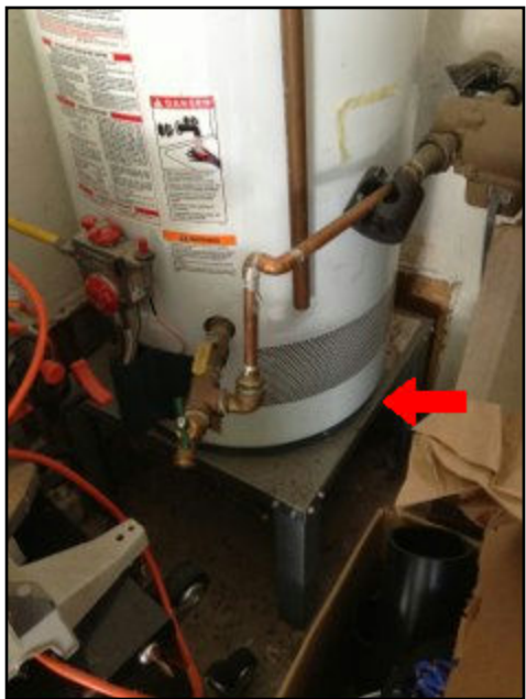
62. Safety pan and drain missing
