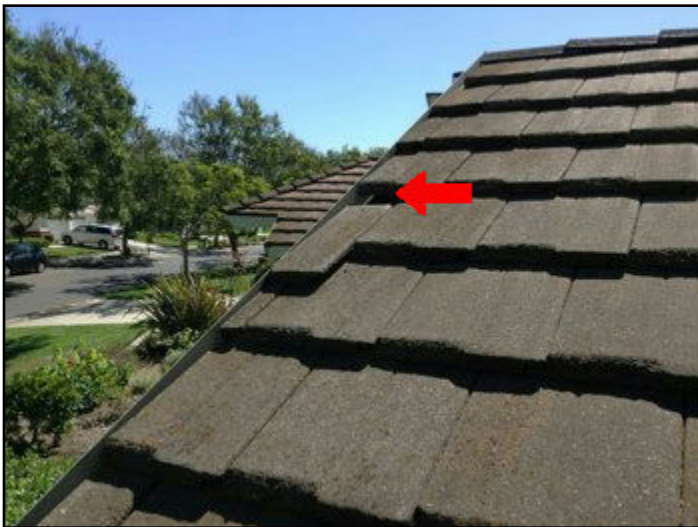
8. Missing, loose or broken pieces
