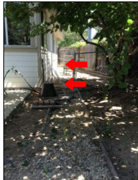
34. Improper slope
