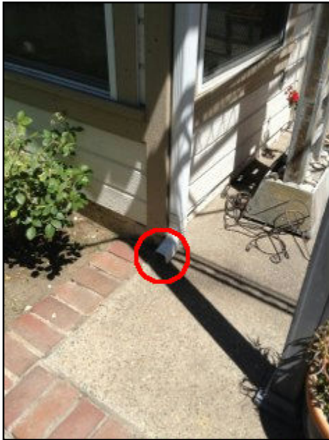
16. Downspouts end too close to building
