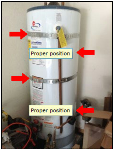
61. Seismic Bracing Incorrect
