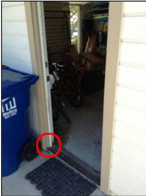
25. Rot or insect damage
