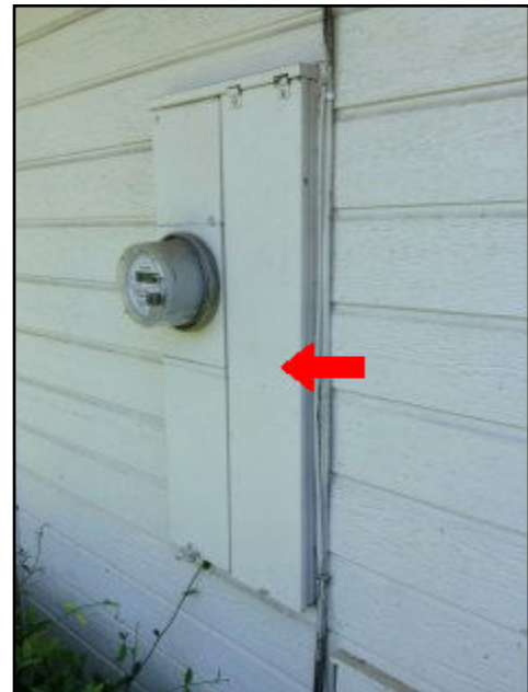
40. Breakers -exterior wall
