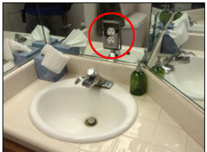
46. Ground Fault Interrupter (GFI) needed
