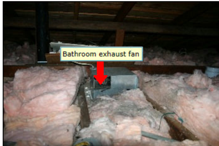
88. Not vented to exterior
