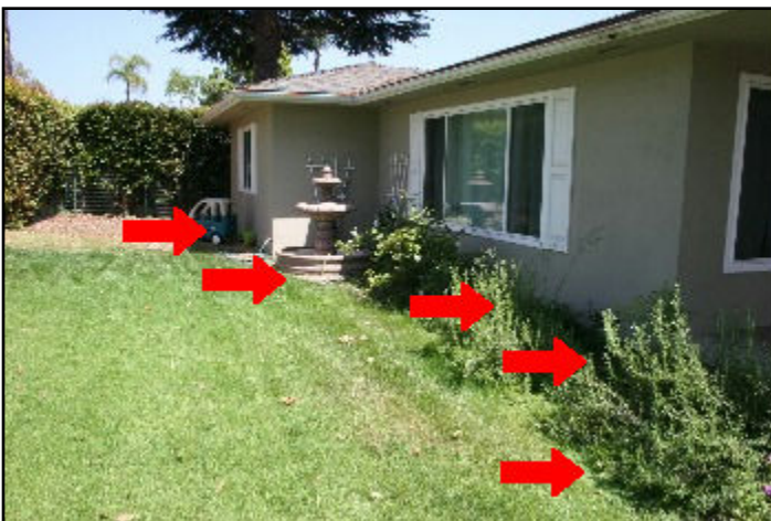
24. Improper slope
