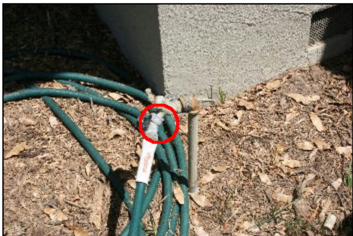
79. Backflow prevention missing
