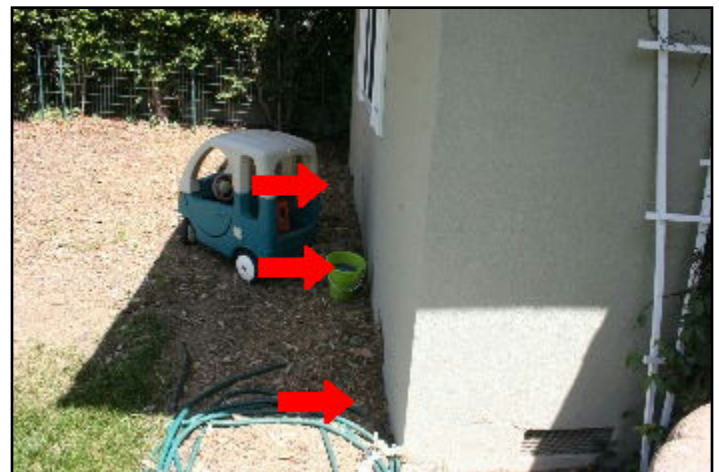
25. Improper slope
