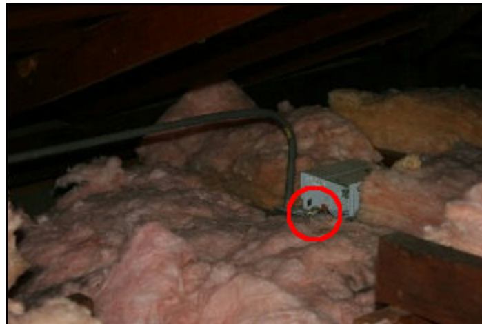
38. Exposed in attics
