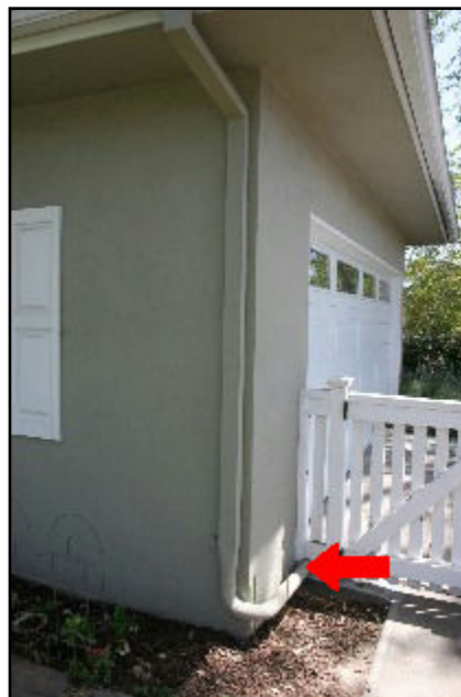
12. Should discharge 6ft. from home
