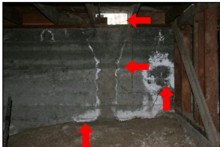
85. Efflorescence
