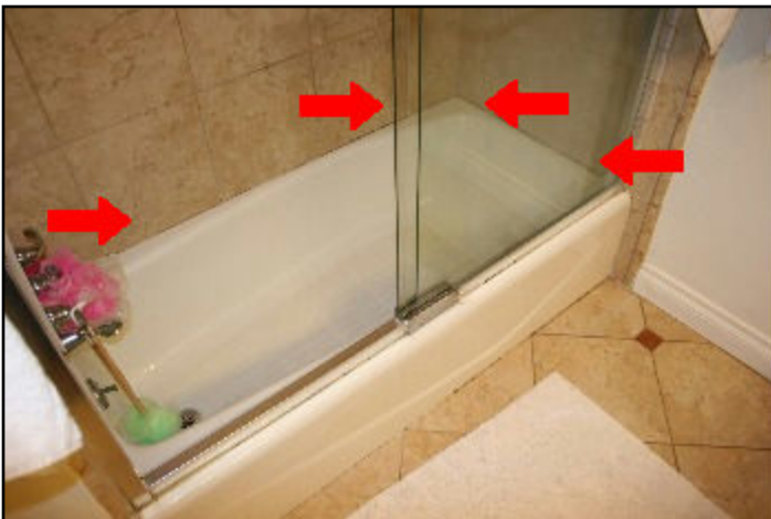
76. Caulking loose, missing or deteriorated
