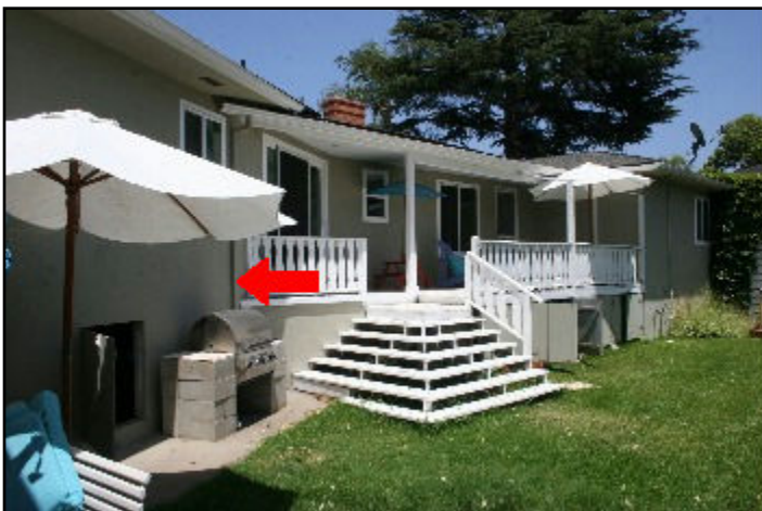
11. Should discharge 6ft. from home
