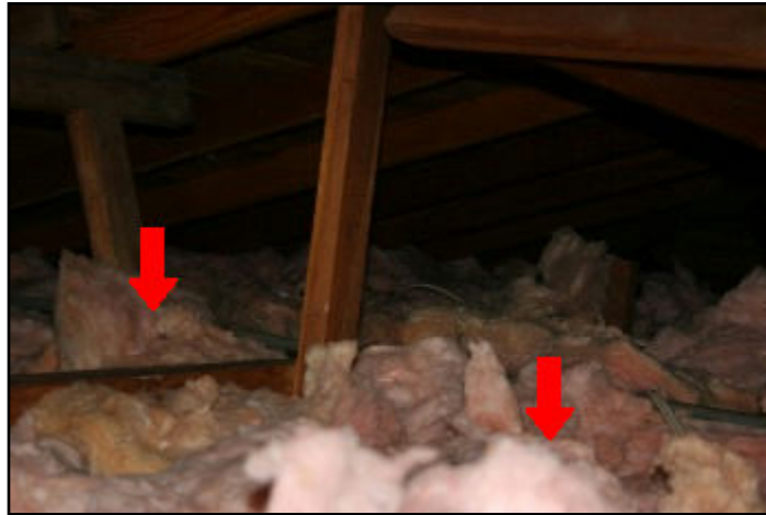
55. Insulation observed in attic space.
