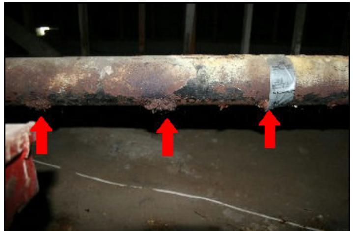
69. Split and damaged
