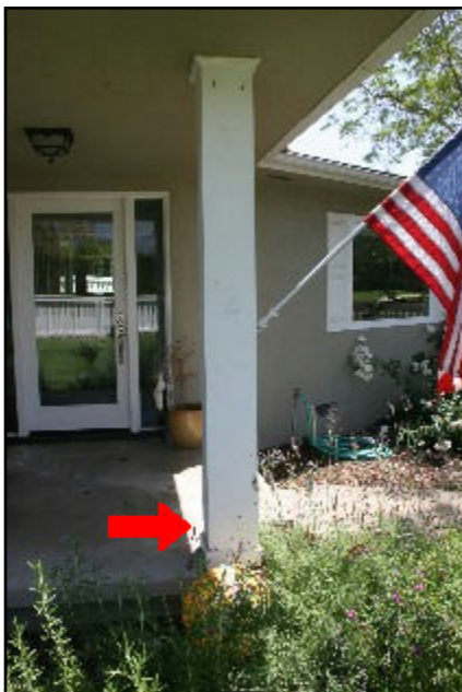
16. Rot or insect damage
