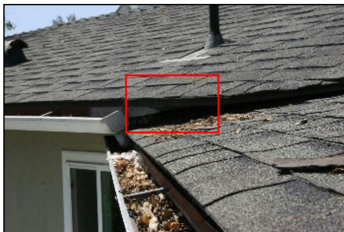
13. Rot or insect damage
