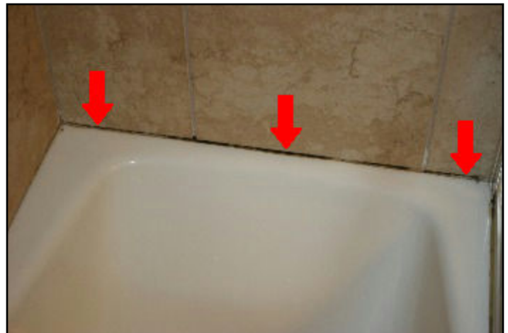
77. Caulking loose, missing or deteriorated
