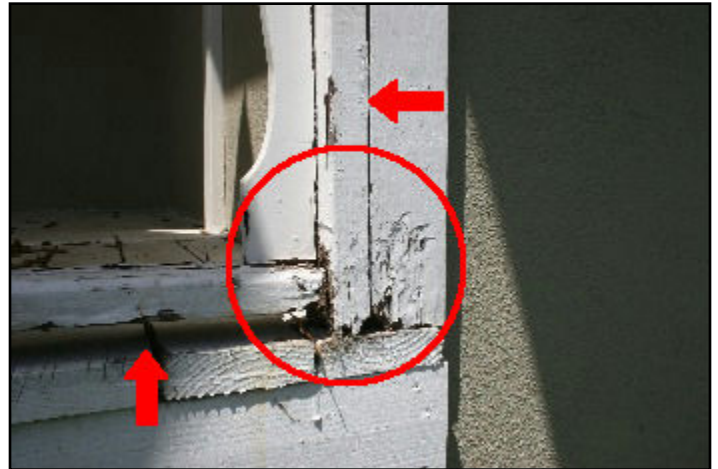
23. Rot or insect damage
