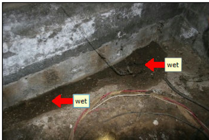
83. Dampness on floor or walls
