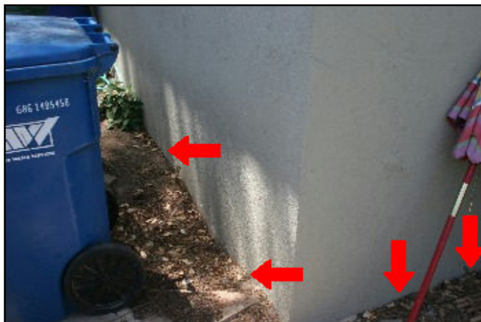
15. No drip screed
