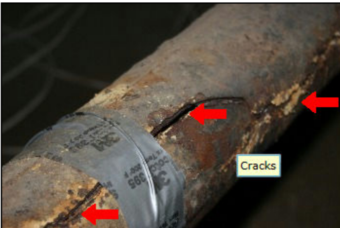
68. Split and damaged
