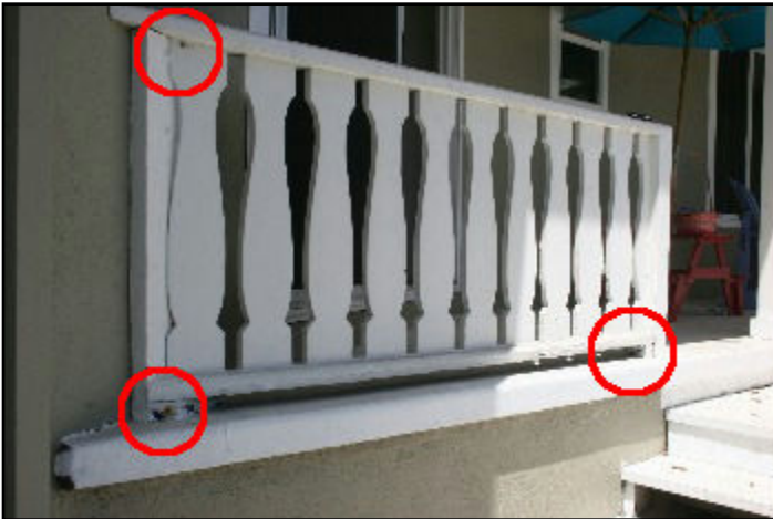
22. Rot or insect damage
