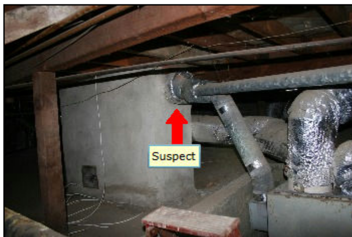
49. Poor connections
