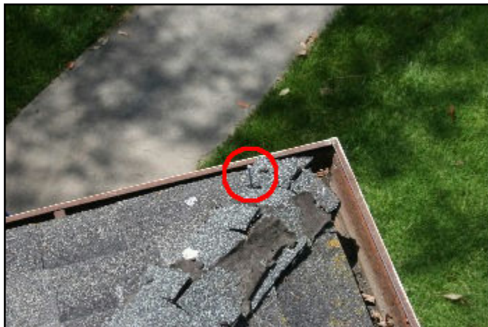
4. Exposed fasteners
