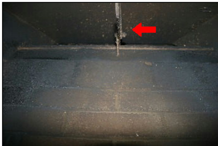
51. Damper in existing fireplace not fixed open
