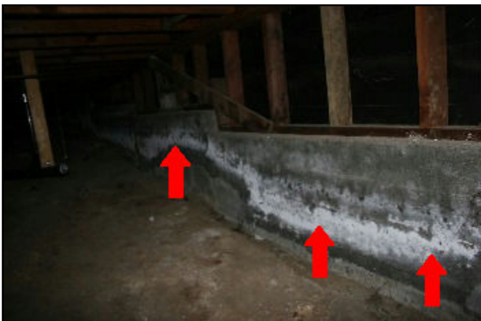
84. Efflorescence
