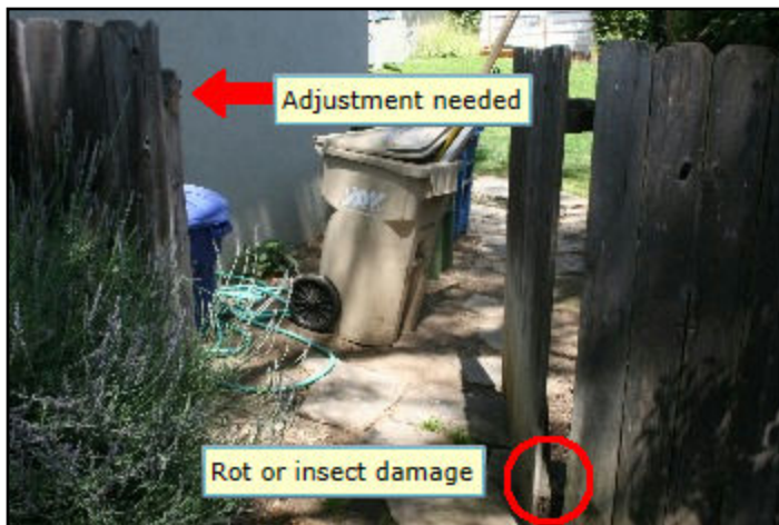
28. Rot or insect damage
