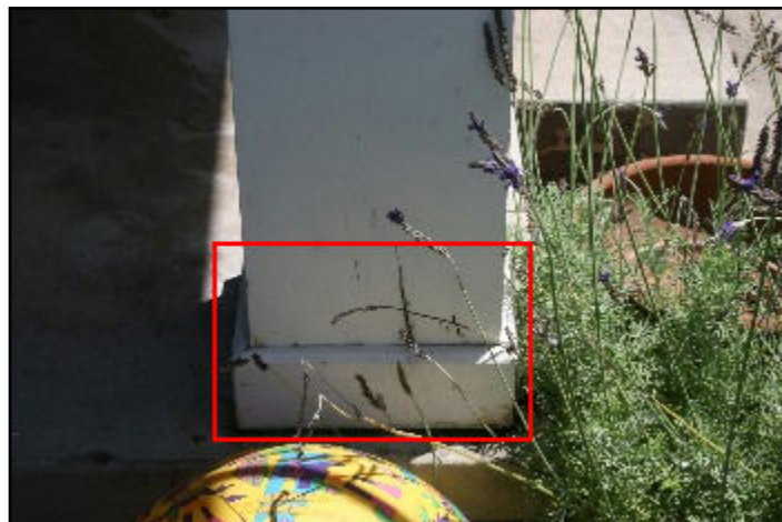
17. Rot or insect damage
