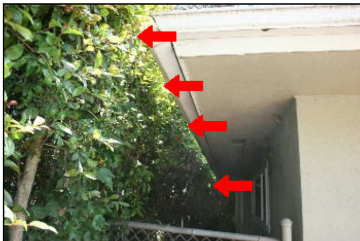
27. Trees or shrubs too close to house
