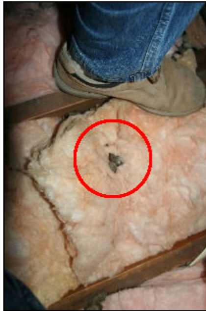
56. Evidence of rodents
