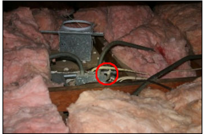
37. Exposed in attics
