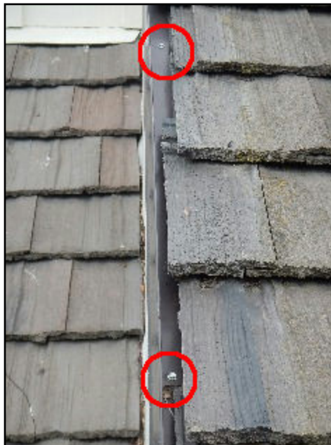
13. Exposed fasteners
