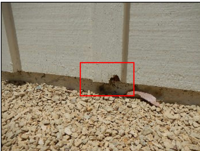
37. Rot or insect damage
