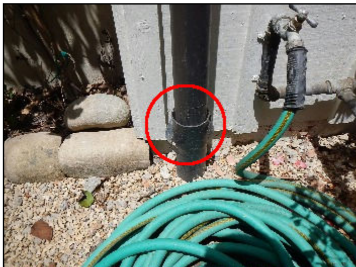
30. Not well secured
