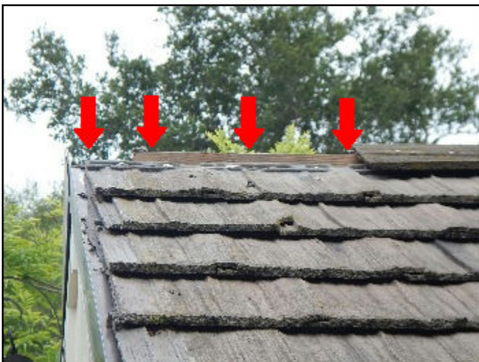
9. Missing or loose hip, ridge, rake, eave...
