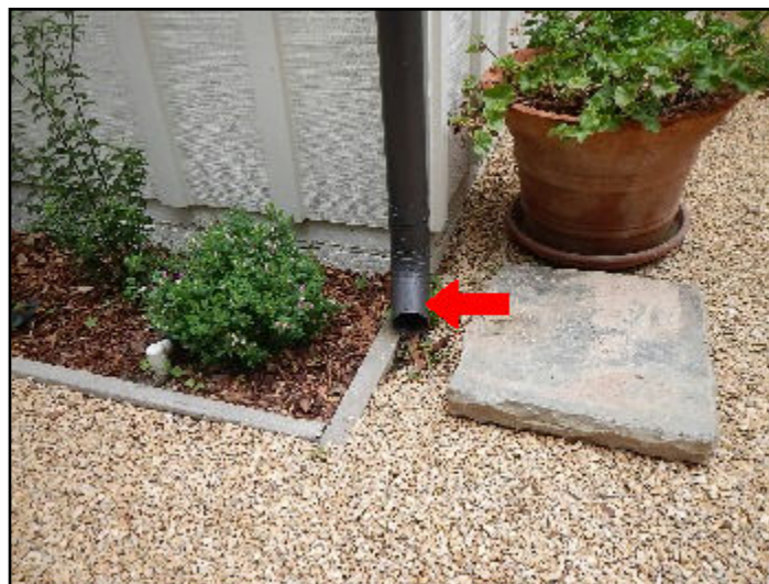
28. Downspouts end too close to building
