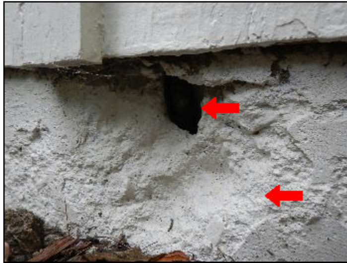
47. Spalling, crumbling or broken material
