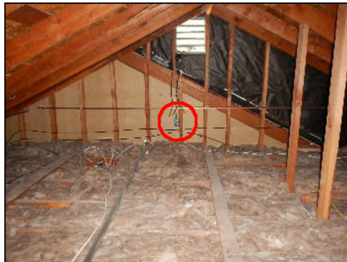
56. Cover loose or missing
