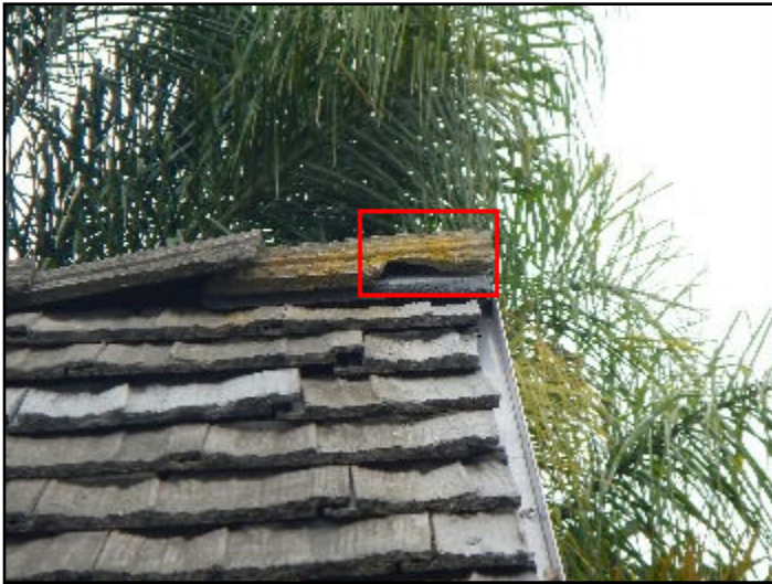
11. Missing or loose hip, ridge, rake, eave...
