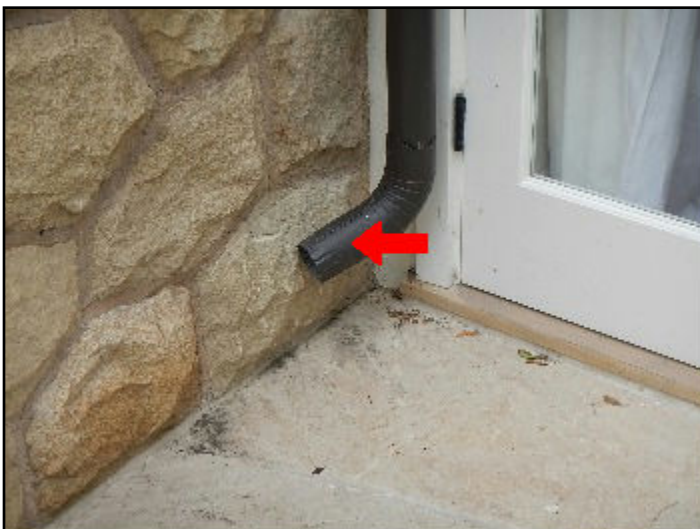
25. Downspouts end too close to building
