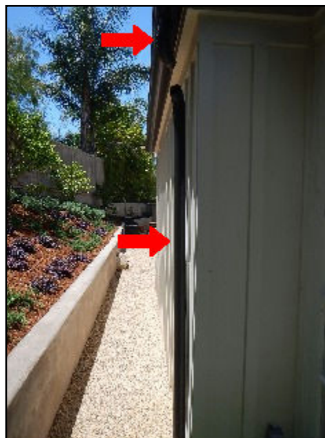
32. Not well secured
