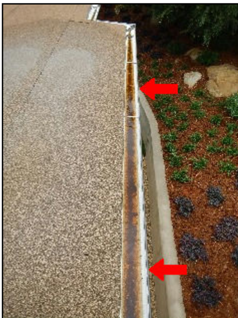
21. Improper slope, ponding
