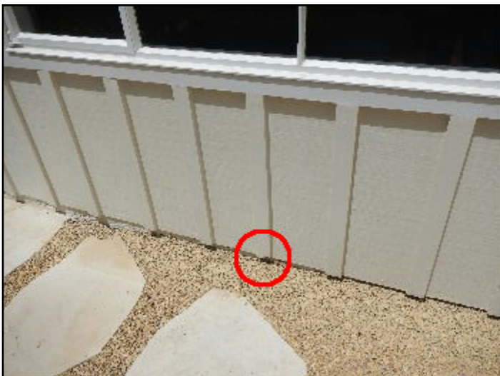
35. Rot or insect damage
