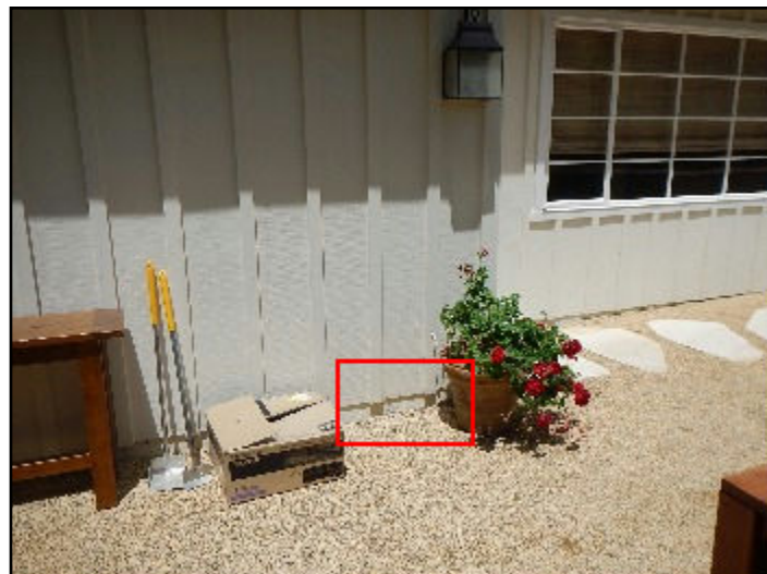
36. Rot or insect damage
