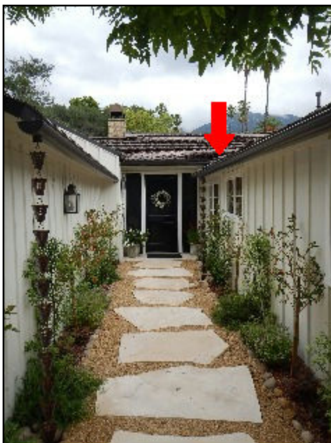
23. Discharging onto roof
