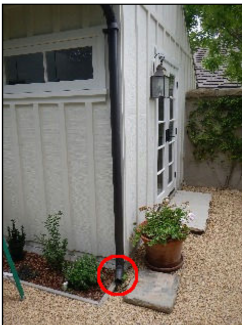
27. Downspouts end too close to building
