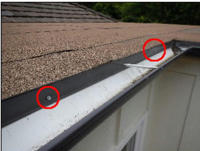
18. Exposed fasteners
