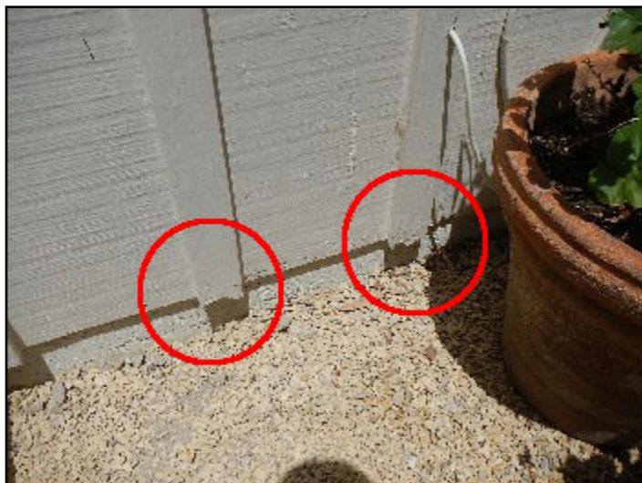
38. Rot or insect damage
