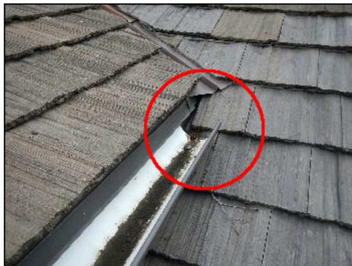
24. Discharging onto roof
