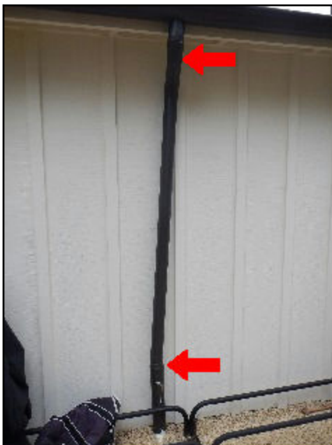
29. Not well secured
