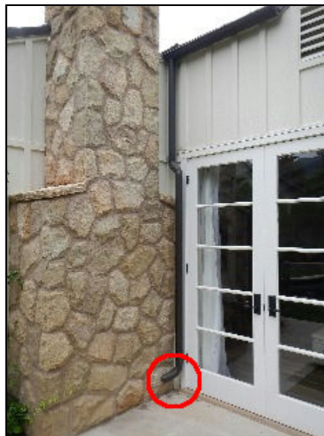
26. Downspouts end too close to building
