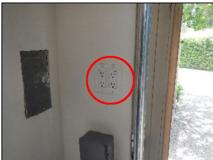
64. Ground Fault Interrupter (GFI) needed
