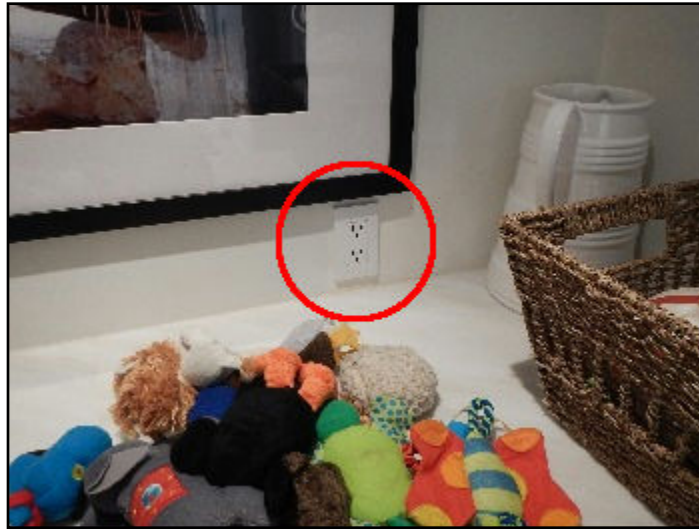
66. Ground Fault Interrupter (GFI) needed
