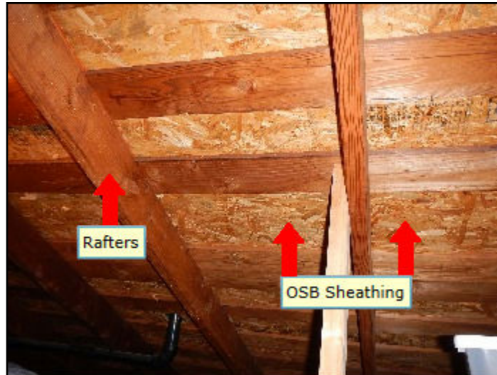
46. Rafters/roof joists
