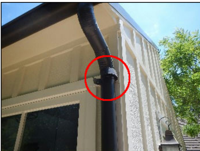
31. Not well secured
