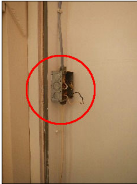
55. Cover loose or missing
