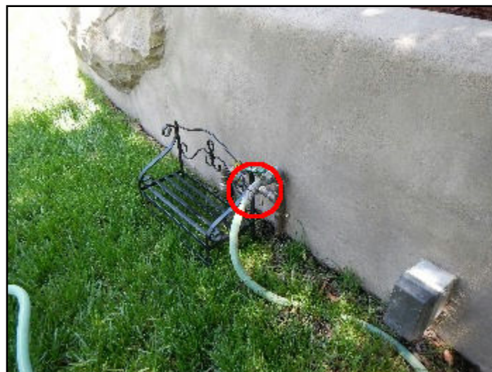
80. Backflow prevention missing
