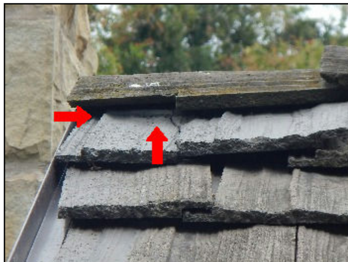
10. Missing or loose hip, ridge, rake, eave...
