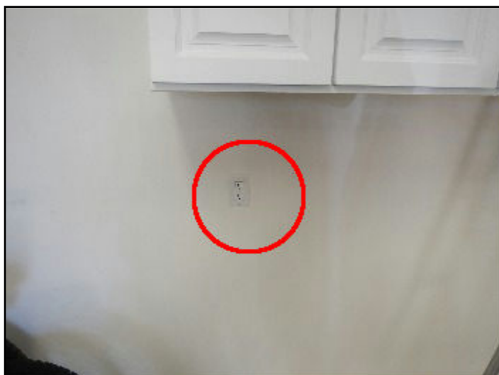
65. Ground Fault Interrupter (GFI) needed
