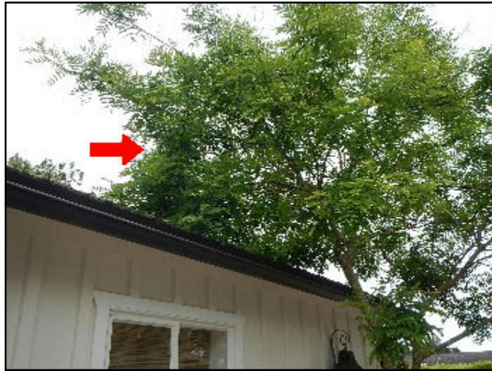
43. Trees or shrubs too close to house
