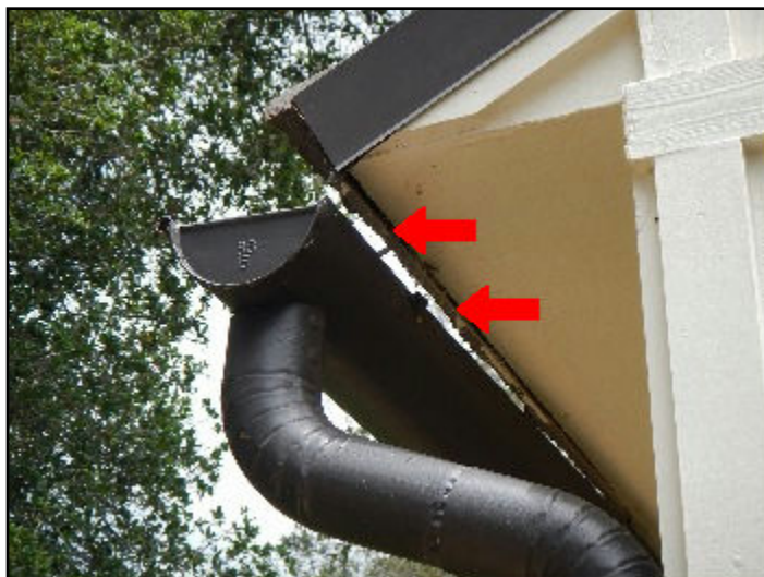
19. Loose or damaged
