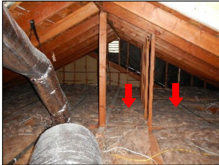
73. Insulation observed in attic space.
