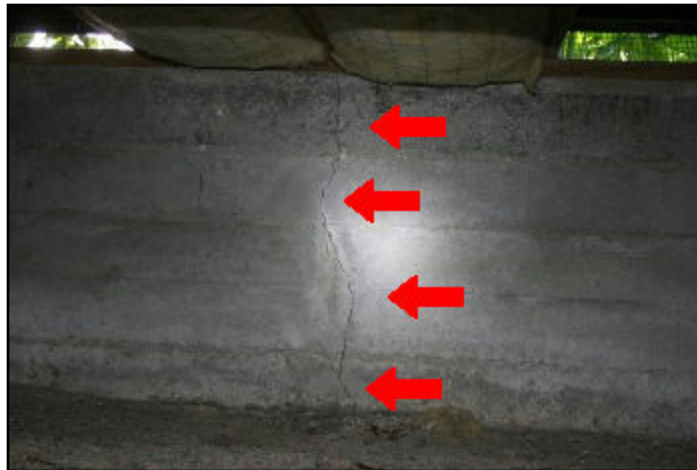
62. Typical minor cracks
