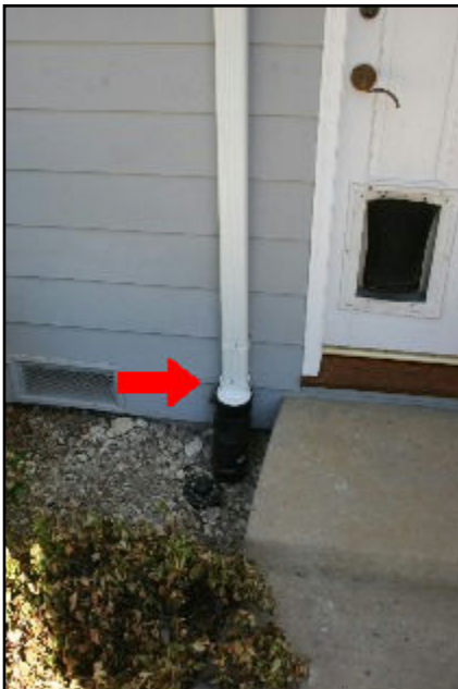
23. Downspouts discharging below grade
