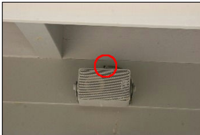
31. Pest intrusion point
