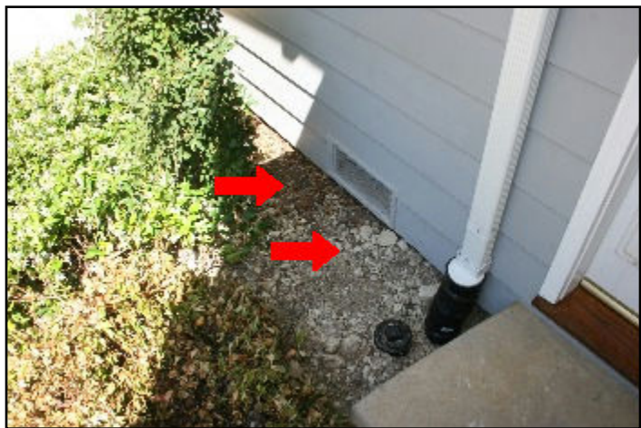
47. Improper slope
