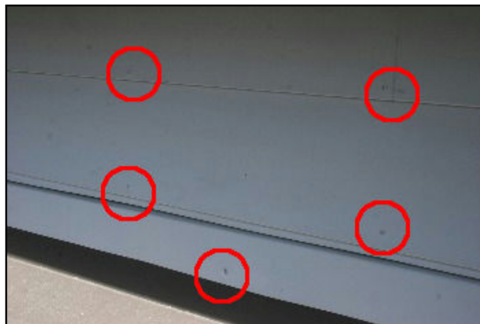
33. Exposed fasteners
