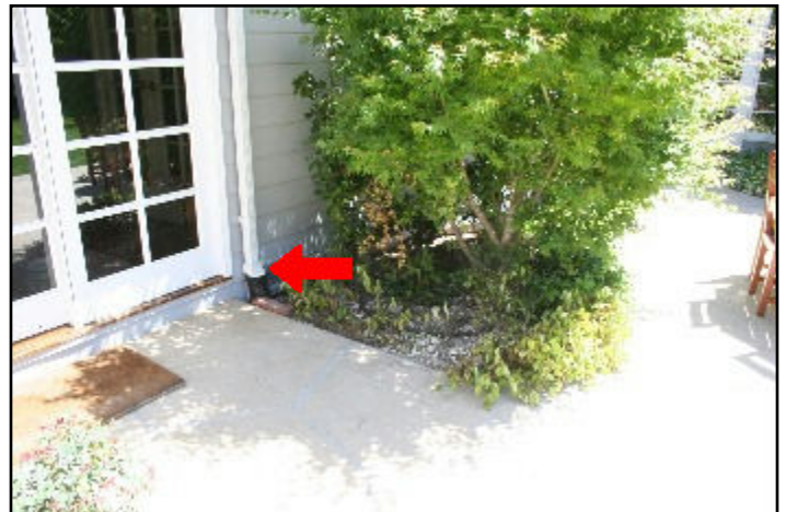
24. Downspouts discharging below grade
