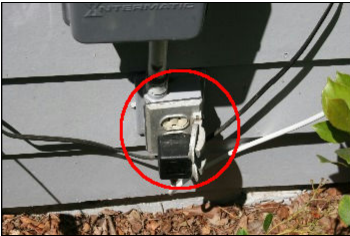
77. Ground Fault Interrupter (GFI) needed
