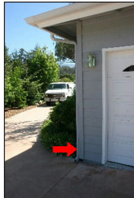
26. Downspouts end too close to building
