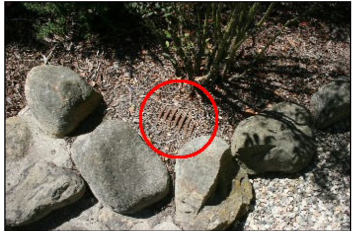
49. Clogged catch basins
