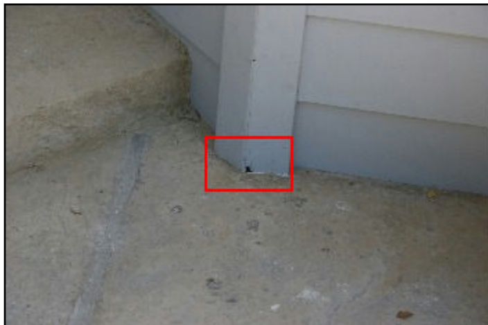
28. Rot or insect damage
