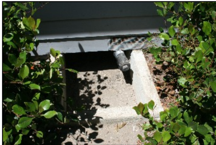
58. Crawl space entry
