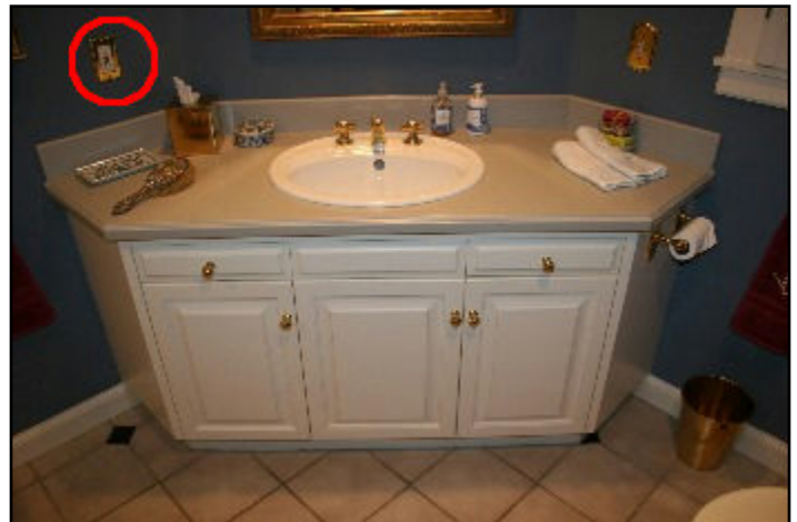
80. GFI test faulty
