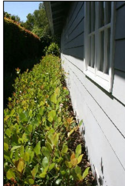
54. Trees or shrubs too close to house
