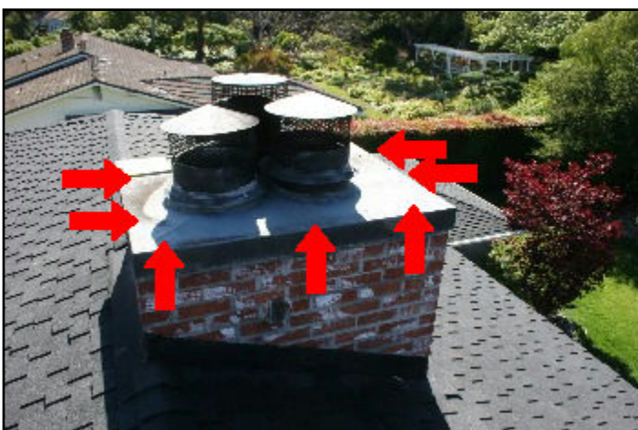
6. Exposed fasteners
