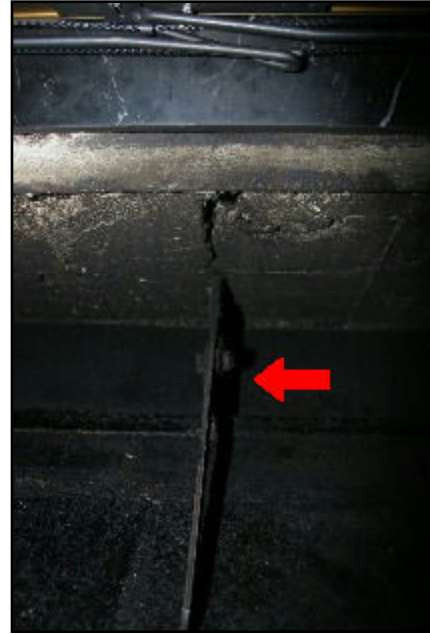
93. Damper in existing fireplace not fixed open
