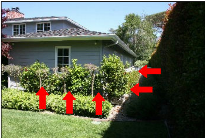
51. Trees or shrubs too close to house
