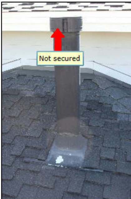
14. Loose or broken vent cap
