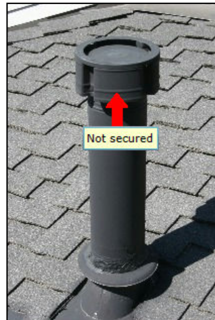
15. Loose or broken vent cap
