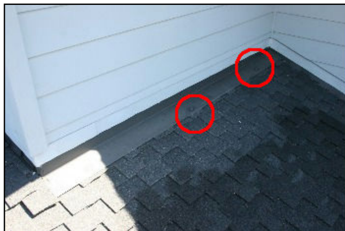
9. Exposed fasteners
