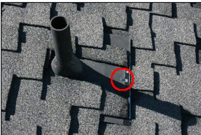
8. Exposed fasteners
