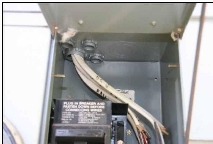
68. Copper - non-metallic sheathed
