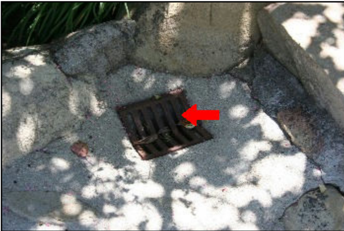
48. Clogged catch basins
