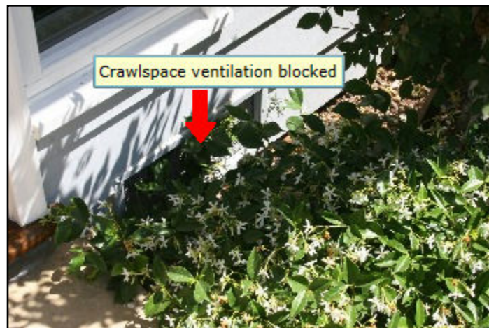
55. Trees or shrubs too close to house
