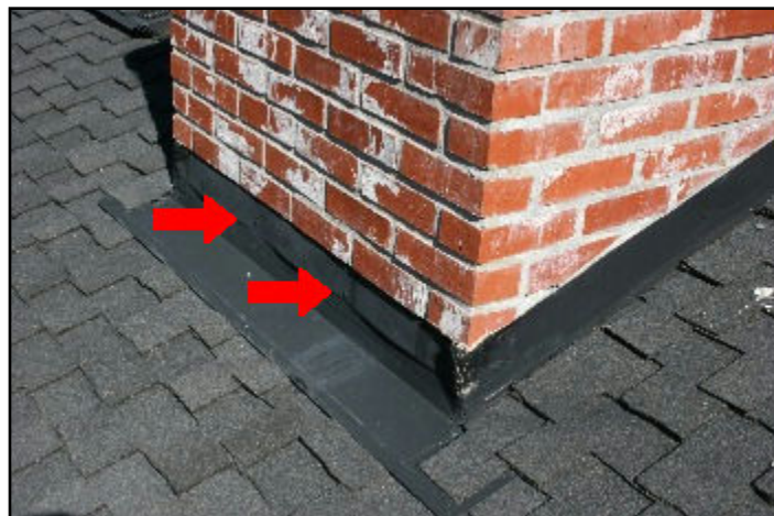
5. Exposed fasteners
