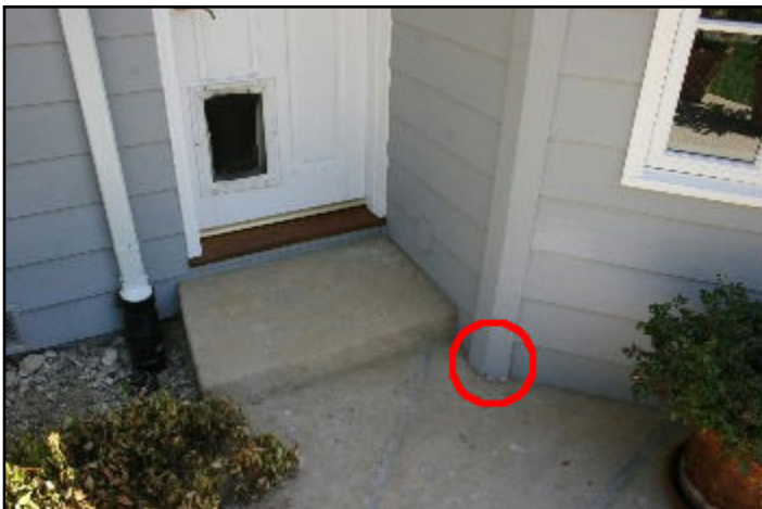
27. Rot or insect damage
