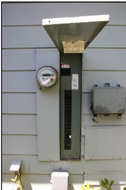
64. Breakers -exterior wall
