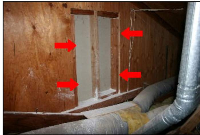
110. Firewall breach
