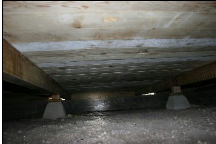
60. Plank subfloor with wooden beams
