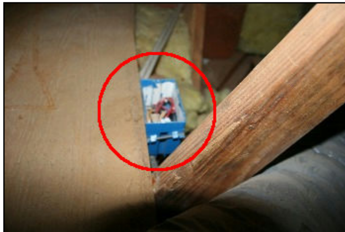
75. Cover loose or missing
