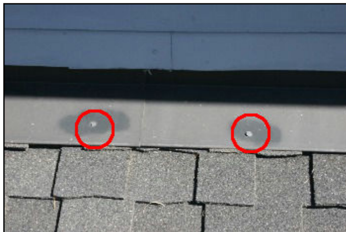
10. Exposed fasteners
