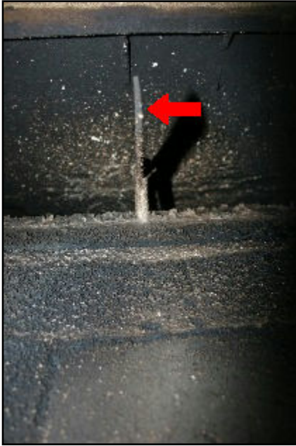
92. Damper in existing fireplace not fixed open
