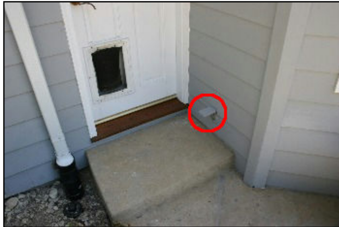
81. GFI test faulty
