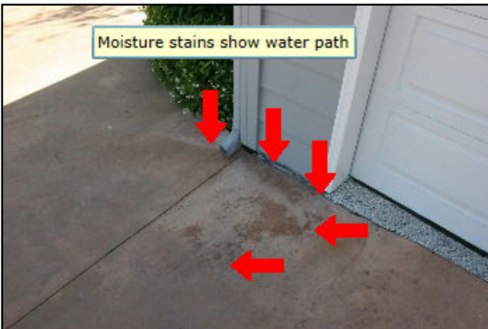
25. Downspouts end too close to building
