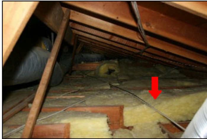
94. Insulation observed in attic space.
