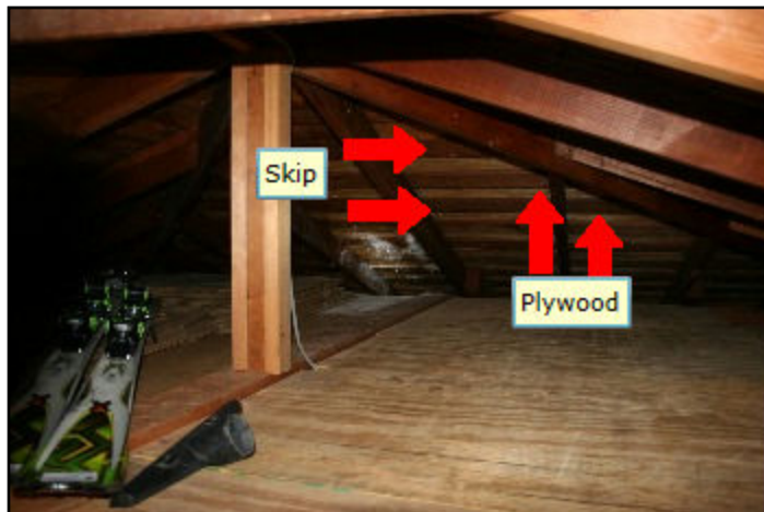
61. Skip and plywood sheathing
