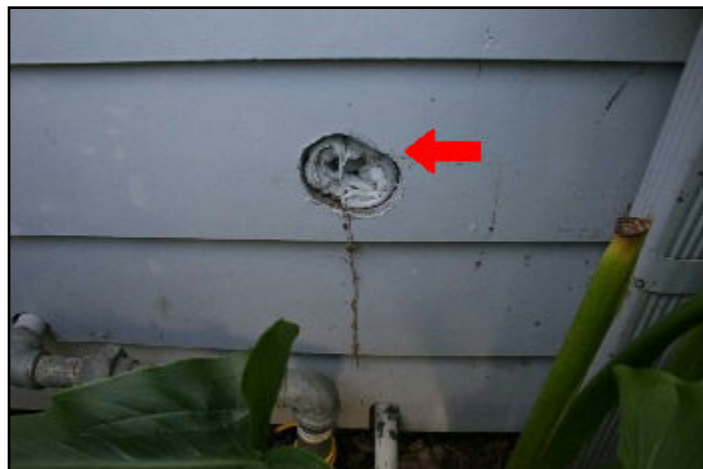
35. Hole in siding
