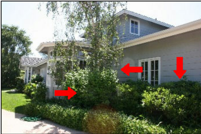
53. Trees or shrubs too close to house
