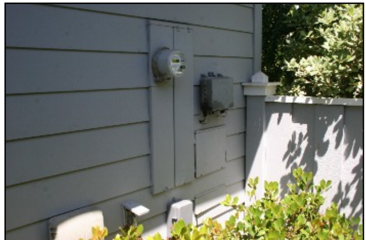
65. Breakers -exterior wall
