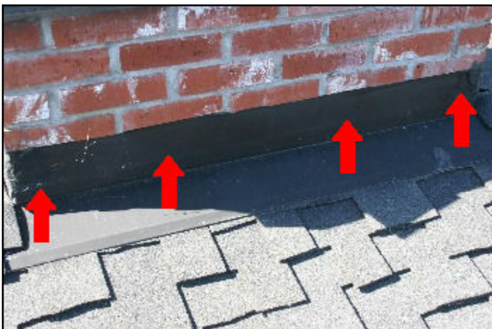
4. Exposed fasteners
