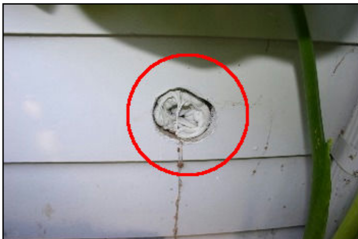
34. Hole in siding
