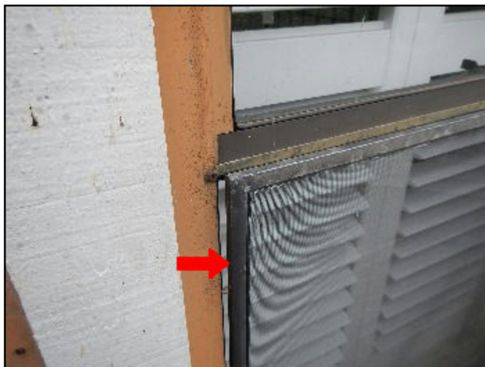
14. Screens broken, torn or missing
