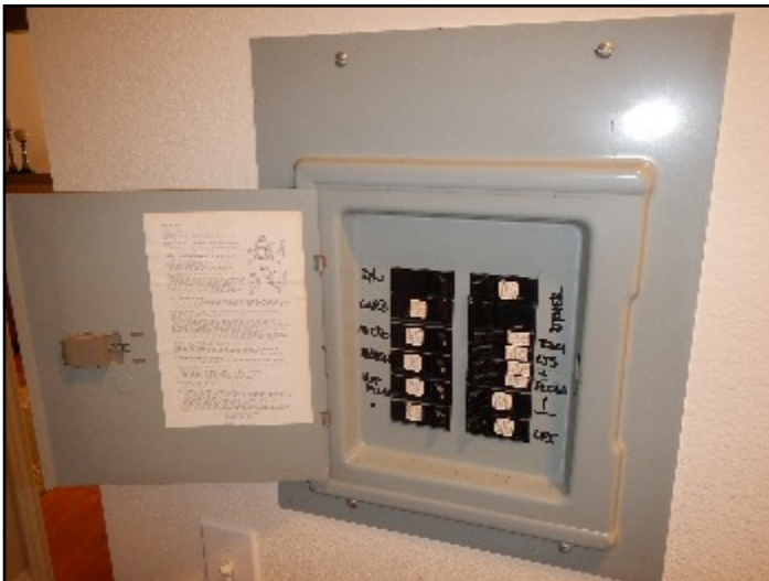
21. Breakers - first floor
