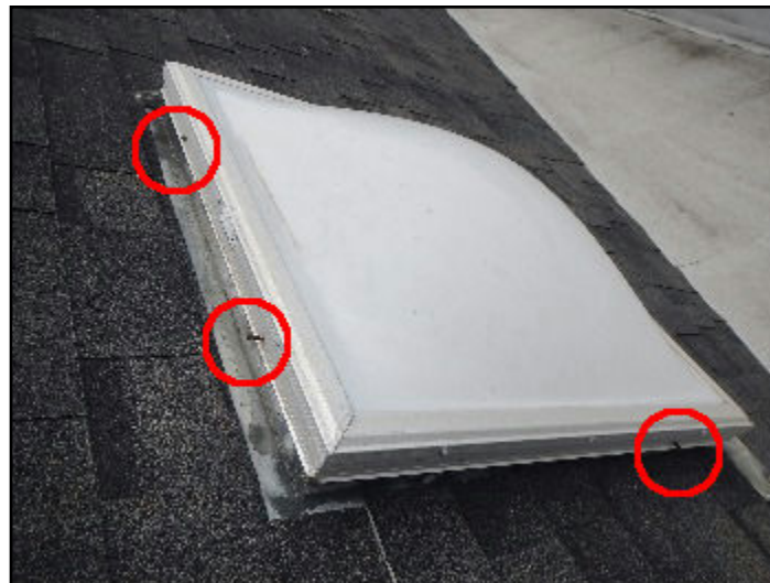
9. Skylight poorly secured to roof
