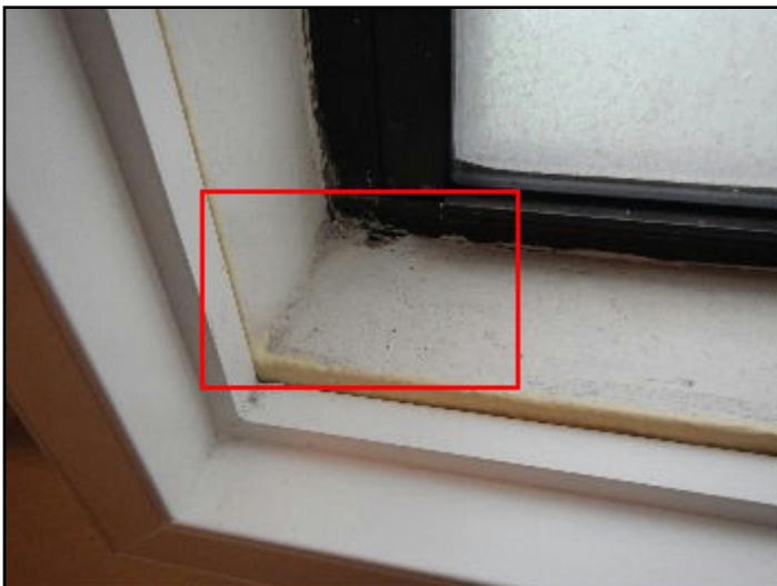
39. Moisture damage
