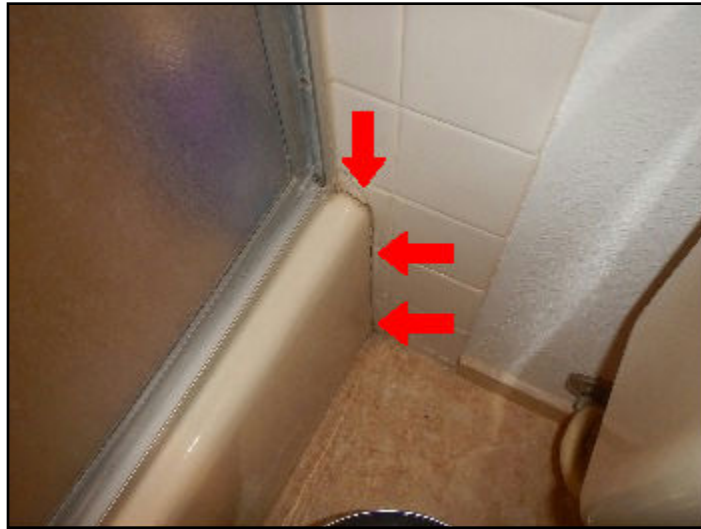
35. Caulking loose, missing or deteriorated
