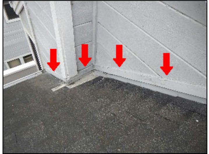
8. Damage, loose, open seams, patched
