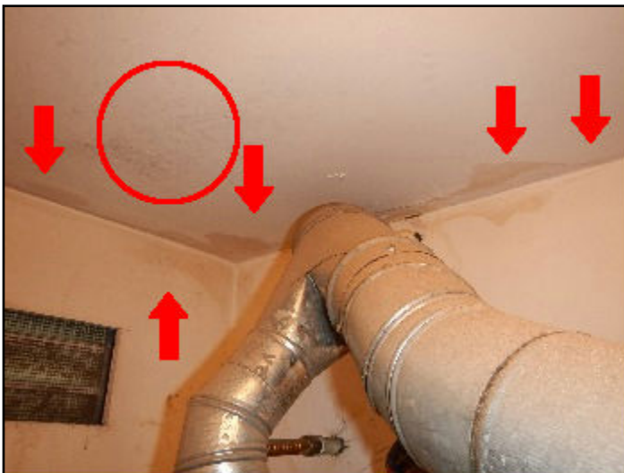
36. Water damage
