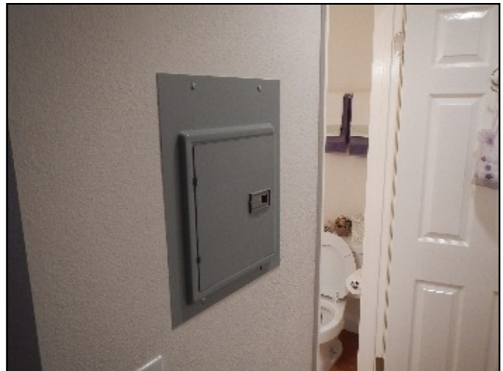
22. Breakers - first floor
