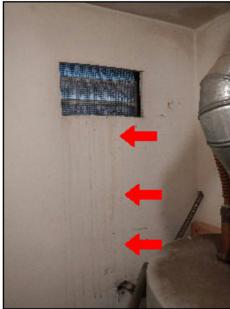
38. Water damage
