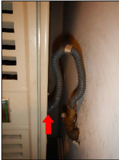
29. Inappropriate materials
