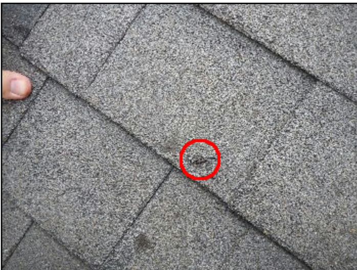
3. Exposed fasteners
