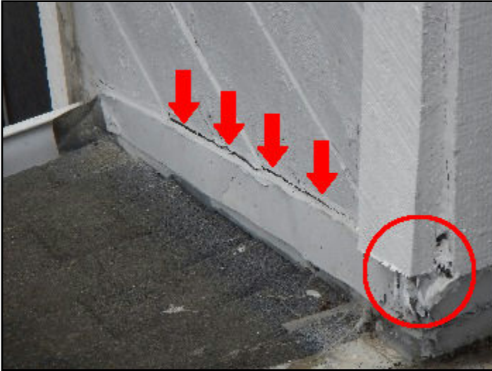
7. Damage, loose, open seams, patched
