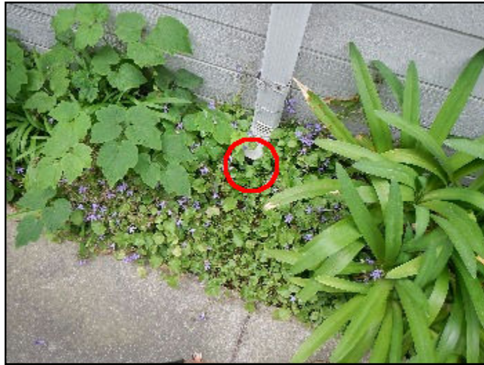
10. Downspouts end too close to building
