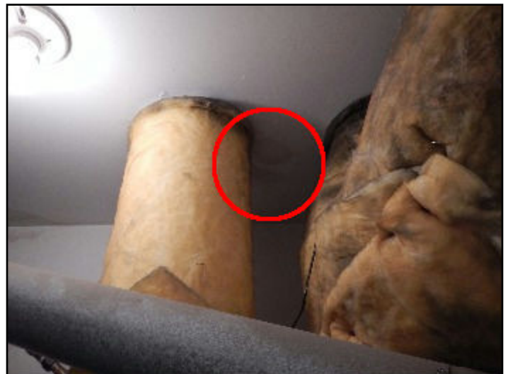
37. Water damage
