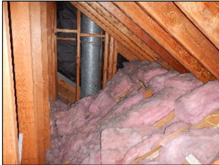
30. Insulation observed in attic space.
