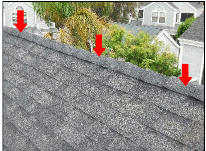
6. Exposed fasteners
