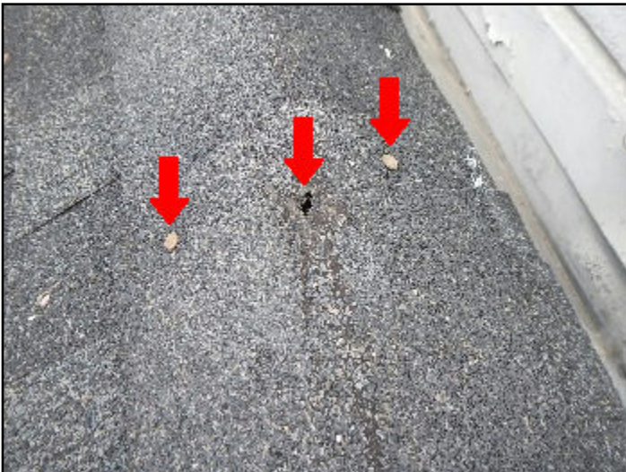
5. Exposed fasteners
