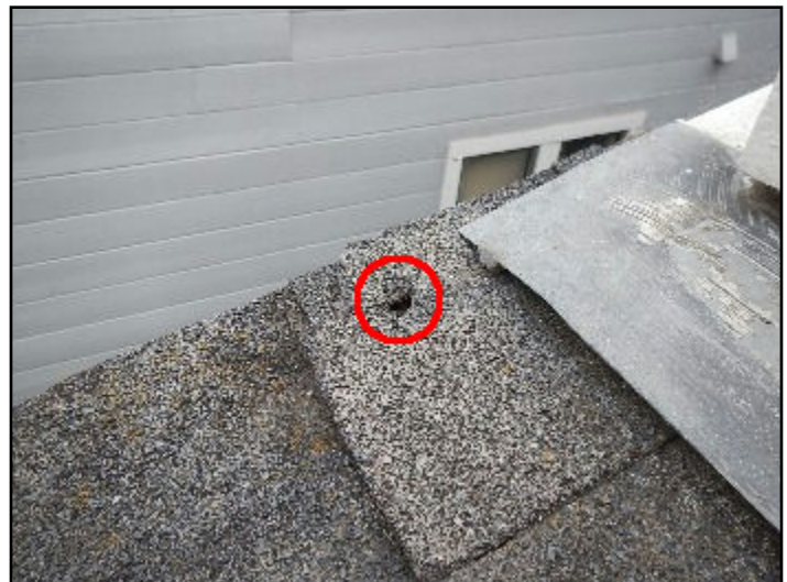
4. Exposed fasteners
