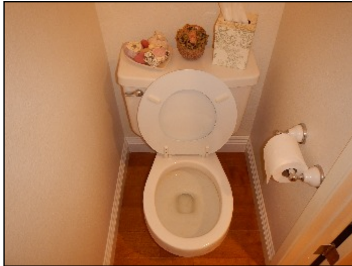
34. Obstructed or weak flush
